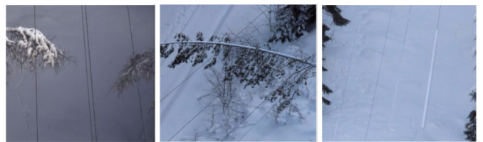
Figure 1: Common faults on power lines (from left to right): trees growing too close to power lines, trees lying across power lines, icing on power lines. In warm countries, icing on power lines may not be a relevant fault; however, in cold countries, such as Norway, it is a very serious problem since thick icing accumulated on power lines can cause a great deal of damage to the lines.
