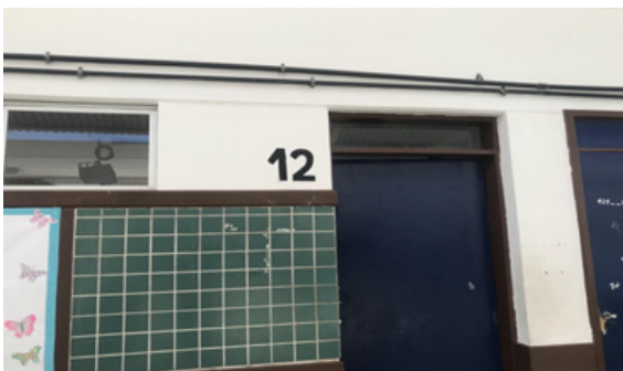
Figure 9 Room 12, third floor - Class - 1902 intervention on the door – during.
