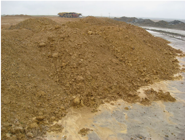
Fig. 2 Soil replacement following coal mining on a reclamation site in southwestern Indiana, USA. Operational procedures in this region call for level grading of the replacement soil followed by planting of native hardwood trees. Photo credit: D.F. Jacobs
