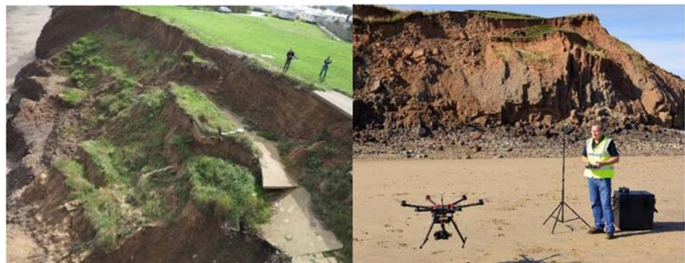
Fig. 9 Coastal cliff landslide surveying using a a DJI “S900” UAV with a digital camera and b a Mikrokopter “Hexakopter XL” (right), Aldbrough, UK (2014), BGS@UKRI[2018].
