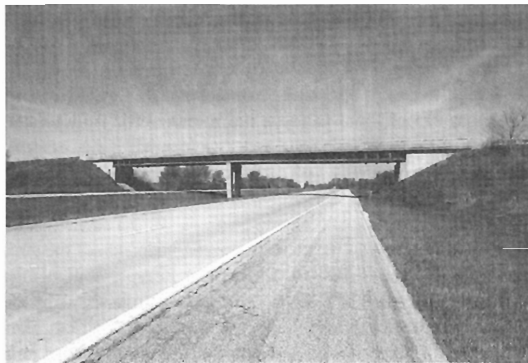
Exhibit 10-3. Typical Grade Separation Structures With Closed Abutments
