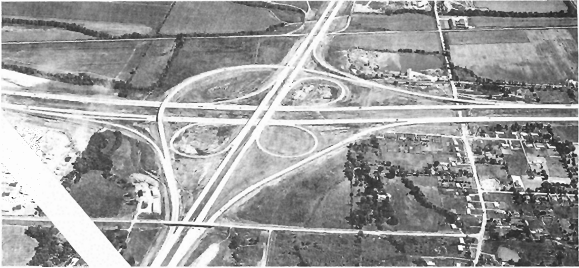
Exhibit 10-40. Four-Leg Interchange, Cloverleaf With a Semidirect Connection
