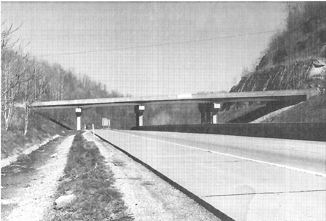
Exhibit 10-4. Typical Grade Separation Structure With Open-End Span
