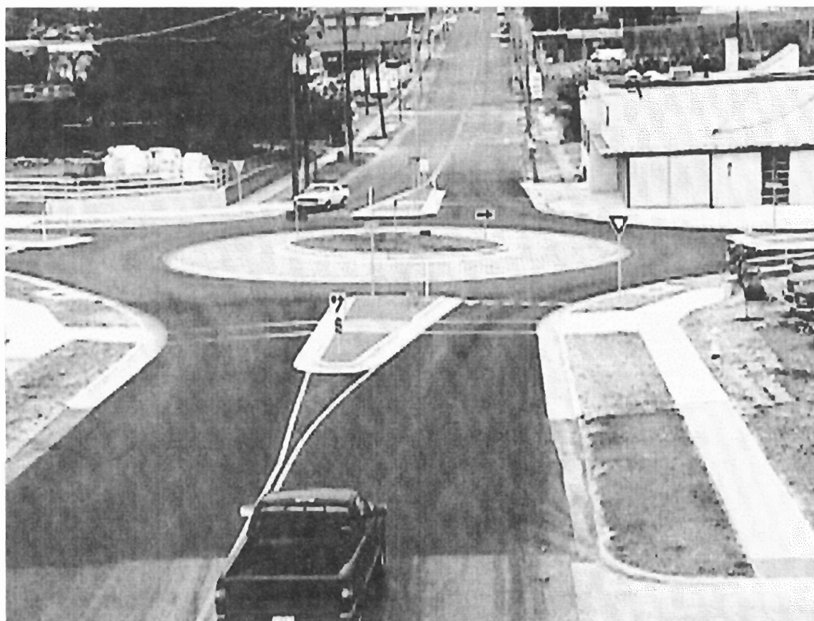
Exhibit 9-16. Typical Modern Roundabout
