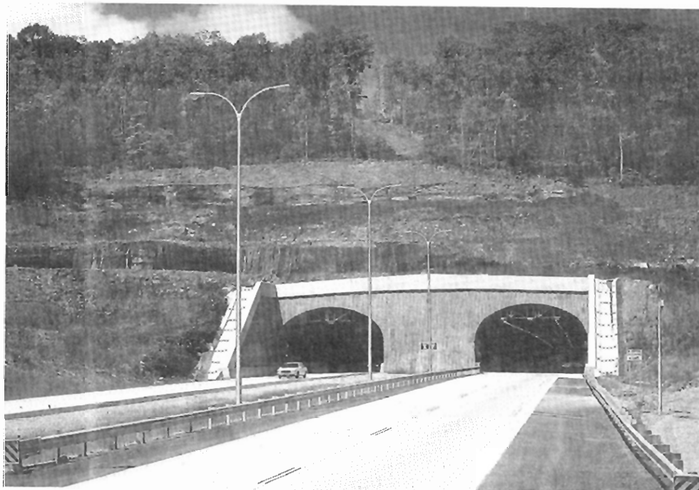
Exhibit 4-19. Entrance to a Freeway Tunnel
