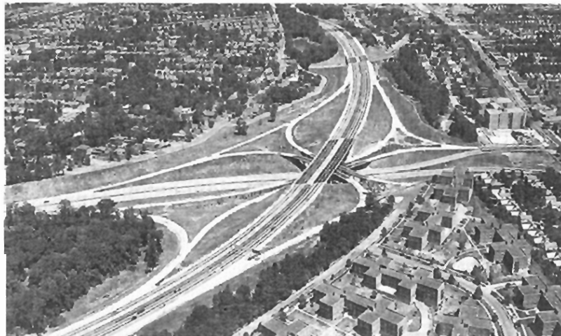
Exhibit 10-35. Four-Level Directional Interchange
