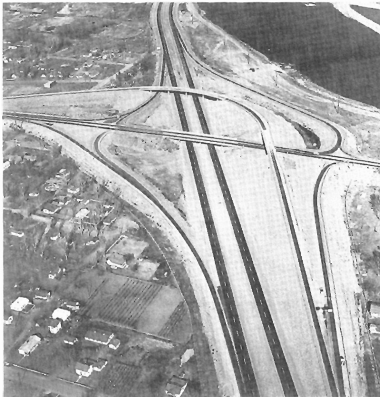
Exhibit 10-39. Four-Leg Interchange, Diamond With a Semidirect Connection
