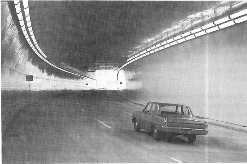
Exhibit 4-20. Interior of a 3-lane One-way Tunnel
