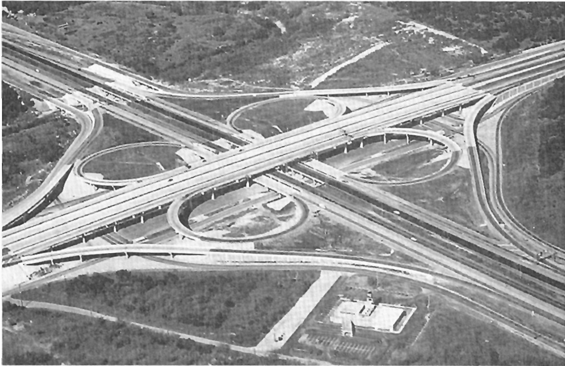
Exhibit 10-42. Freeway with a Three-Level Cloverleaf Interchange
