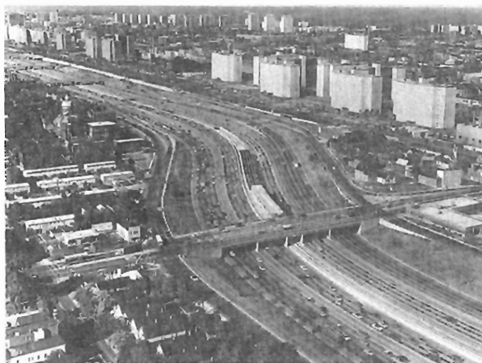
Exhibit 8-25. Dual-Divided Freeway With a 4-3-3-4 Roadway Arrangement
