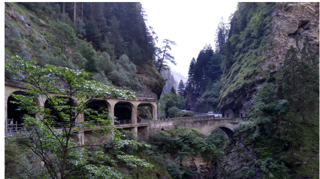
Figure 1: Rockfall protection structures and bridges in a 300 m deep gorge (Viamala, Thusis, Switzerland), where the GNSS reception is absent or unreliable for autonomous UAV guidance.
