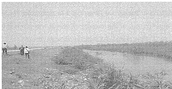
Figure 4. 5km of seadyke protected by mangroves in Thai Do commune and therefore, not eroded in presence of the storm Damrey (Photo: Phan Hong Anh taken on 10/10/2005)
