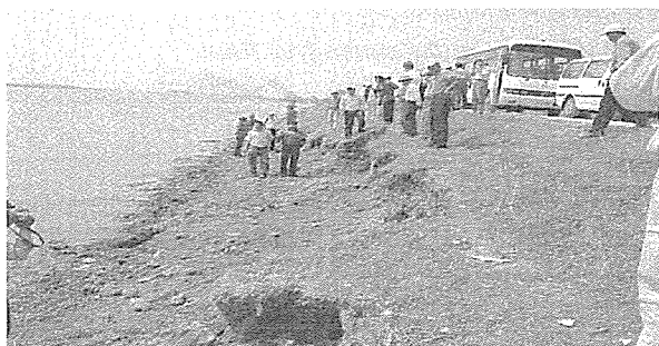
Figure 3. 650m of central seadyke in Tan Boi village, Thai Do commune, Thai Thuy district, Thai Binh province eroded due to storm Damrey (No 7) as a result of mangrove absence (Photo: Phan Hong Anh taken on 10/10/2005)
