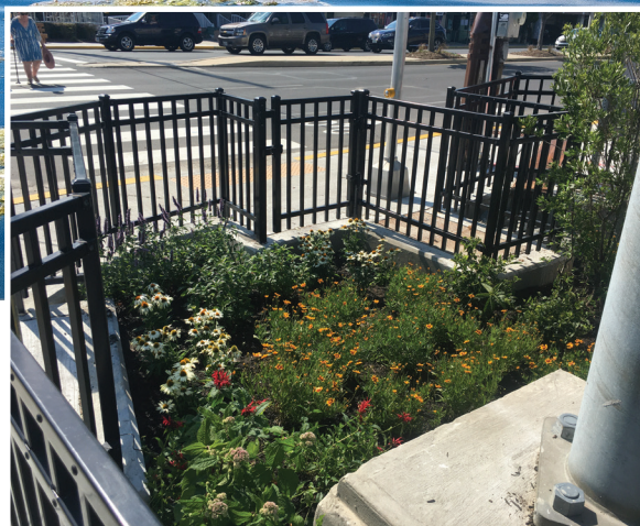
Bioretention facility installed on Read Avenue, Dewey Beach, in 2020.
