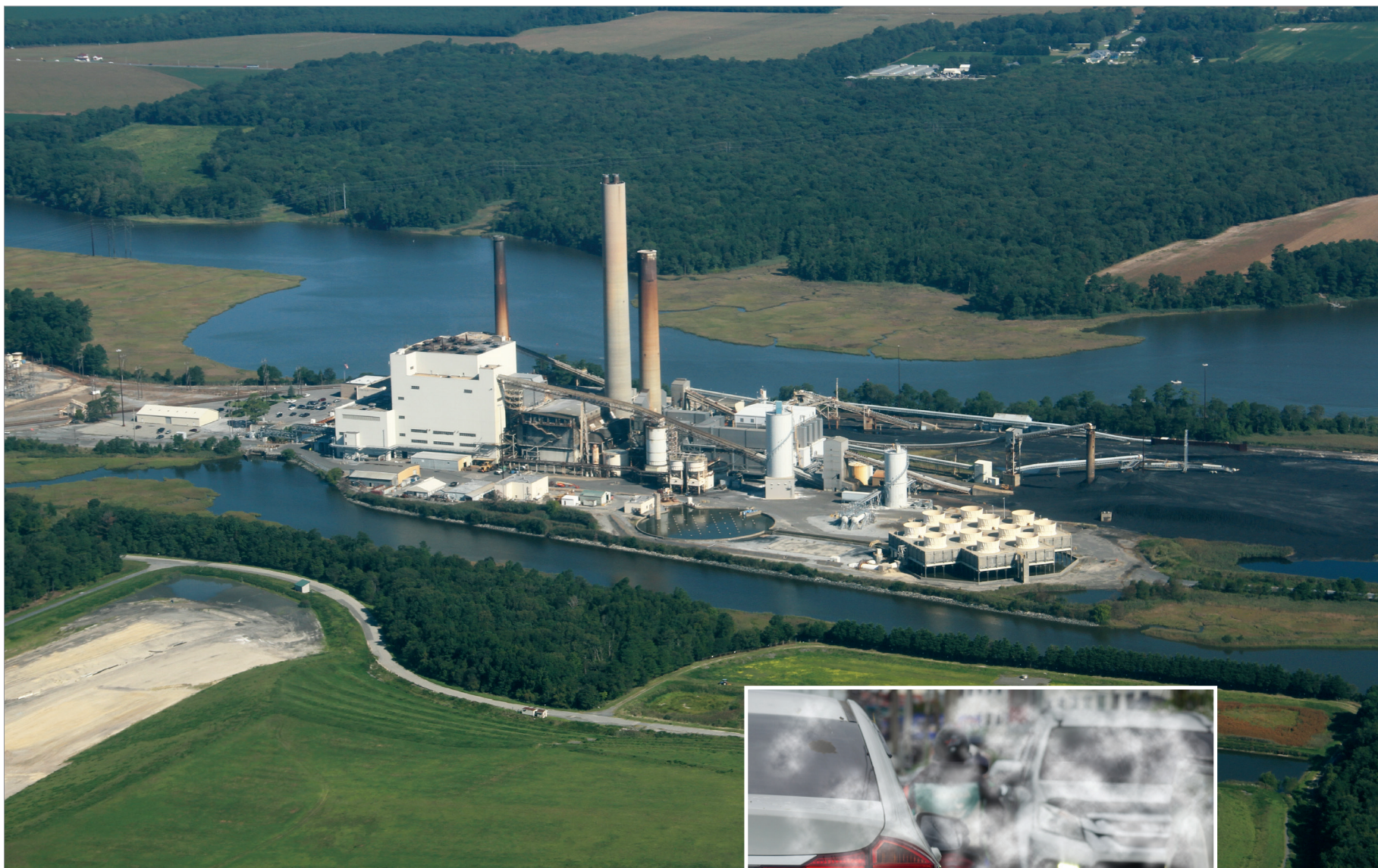
In 2009 and 2011, the NRG power plant in Millsboro was upgraded to meet higher emission standards.
