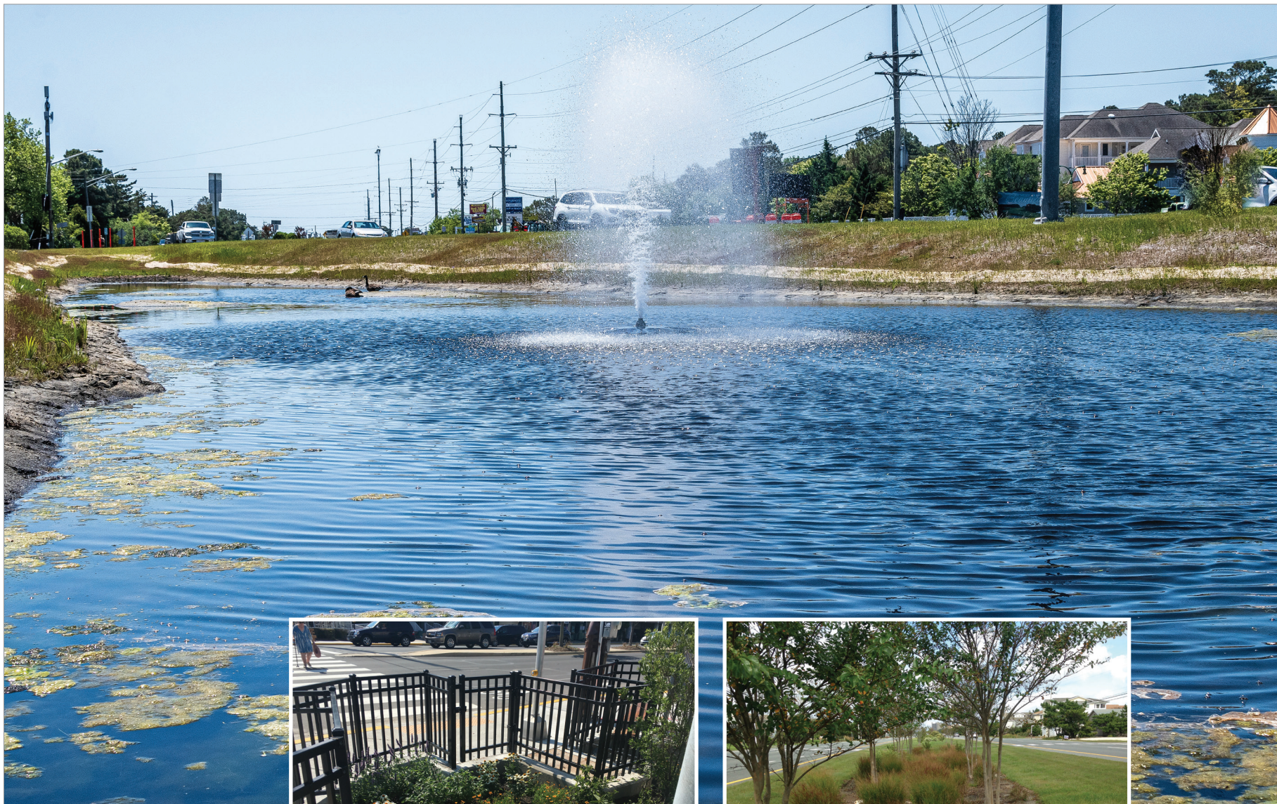
The Anchorage Canal Drainage Area Retrofit Project installed a suite of practices to restore water quality in Bethany Beach and South Bethany, including this stormwater pond and wetland constructed in 2021.
