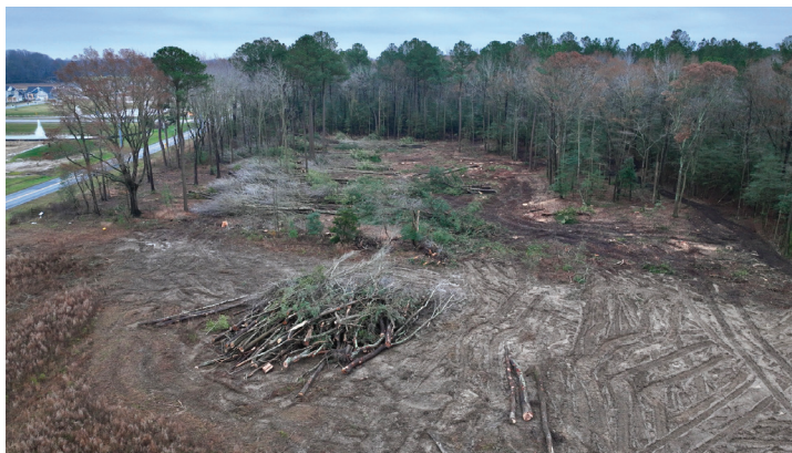
Tree removal for development near Love Creek.
