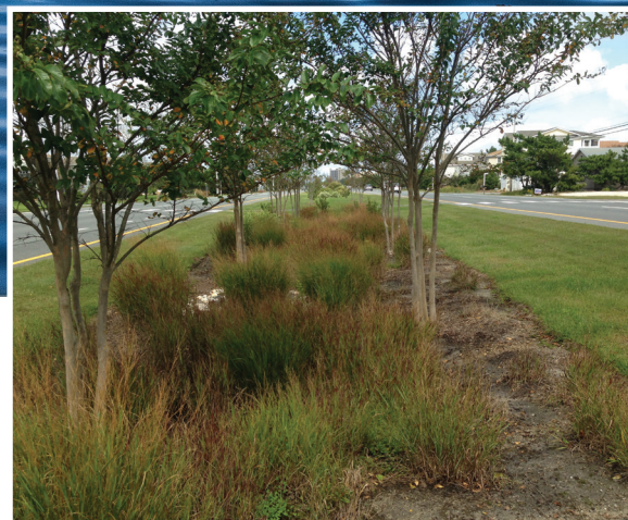
Bioretention retrofit installed in the median of Coastal Highway in South Bethany.
