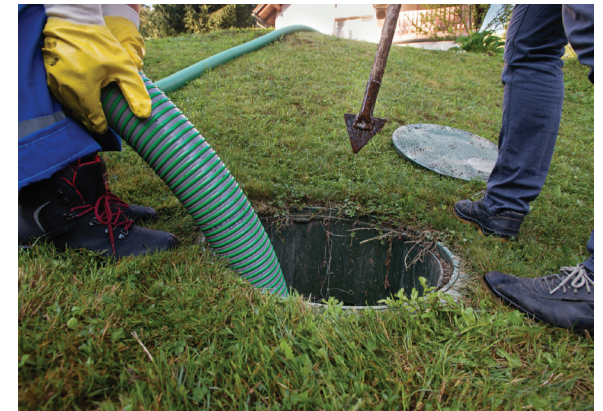
Pumping a septic tank.
