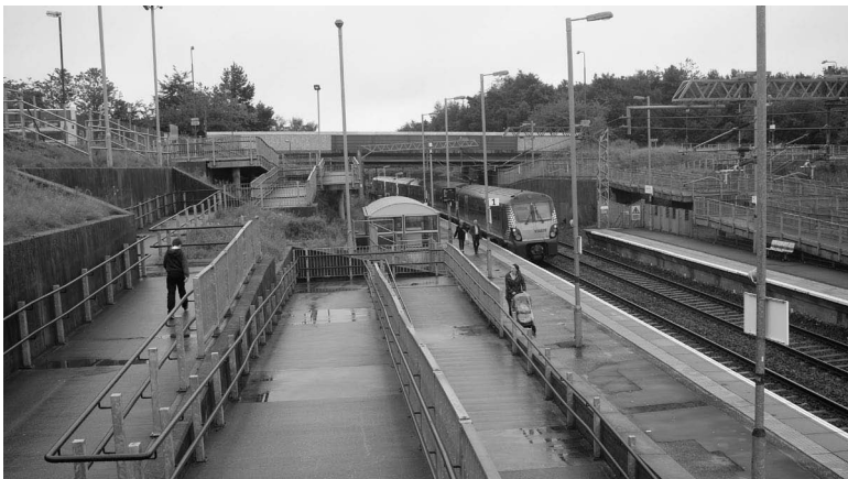
FIGURE 22.4 An “accessible” route to the platform.
