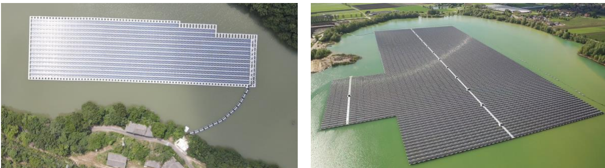
Figure 2: Aerial pictures of both floating PV systems (left: FPV_A, right: FPV_B).
