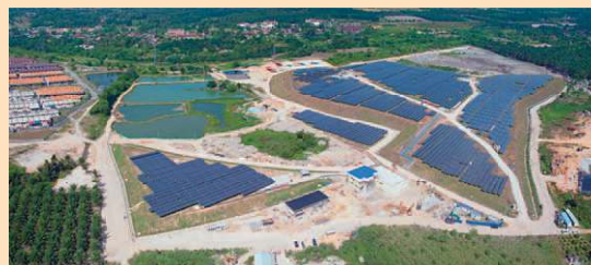
8 MW PV on landfill, Pajam, Malaysia
