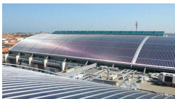
Green Utility SpA-owned Si-a 4,3 MWp PV plant, Rimini Fair, by the contractor Acea Arse SpA
