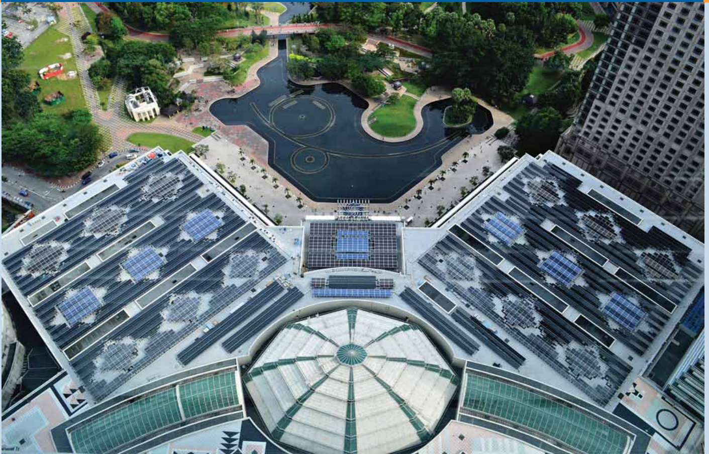
Fig. 2 - 685 kW Solar PV at SURIA KLCC (Shopping Mall), Malaysia (Photo: PETRONAS).
