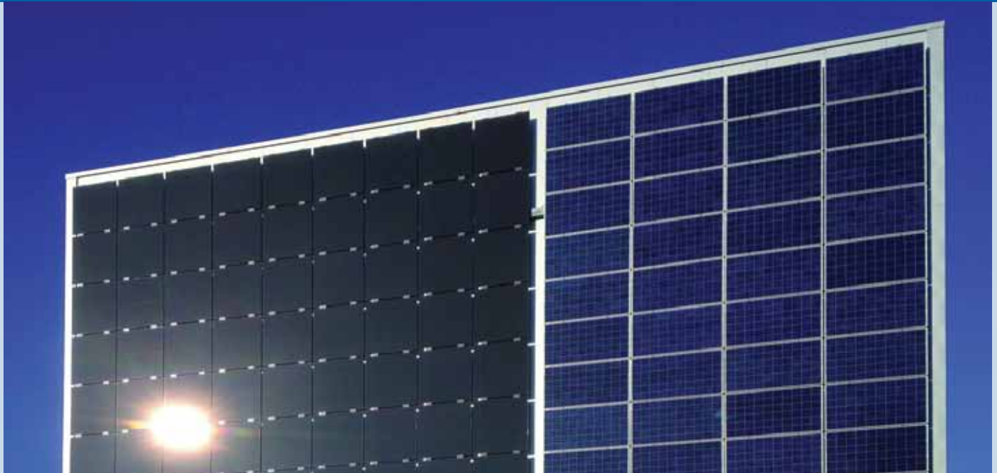
Fig. 1 - PV façade with micromorphous silicon (left, 10,8 kW) and multicrystalline silicon PV modules (right, 11,3 kW) (system development and photo: Jansen).
