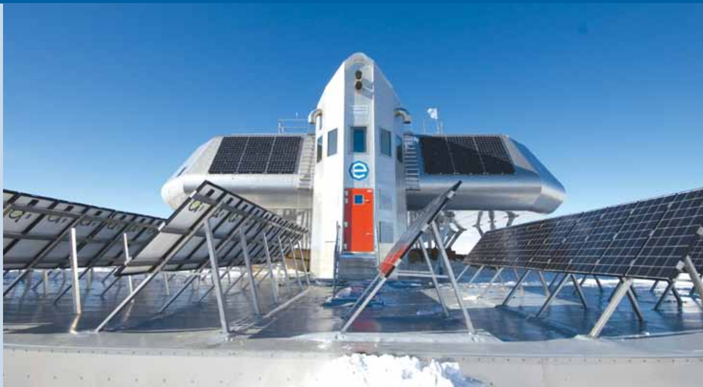
Fig. 1 - Polar Station: the Belgian Queen Elisabeth Station is the first zero emission polar station and was built in 2007-2008. Wind and solar power are the only energy sources.
