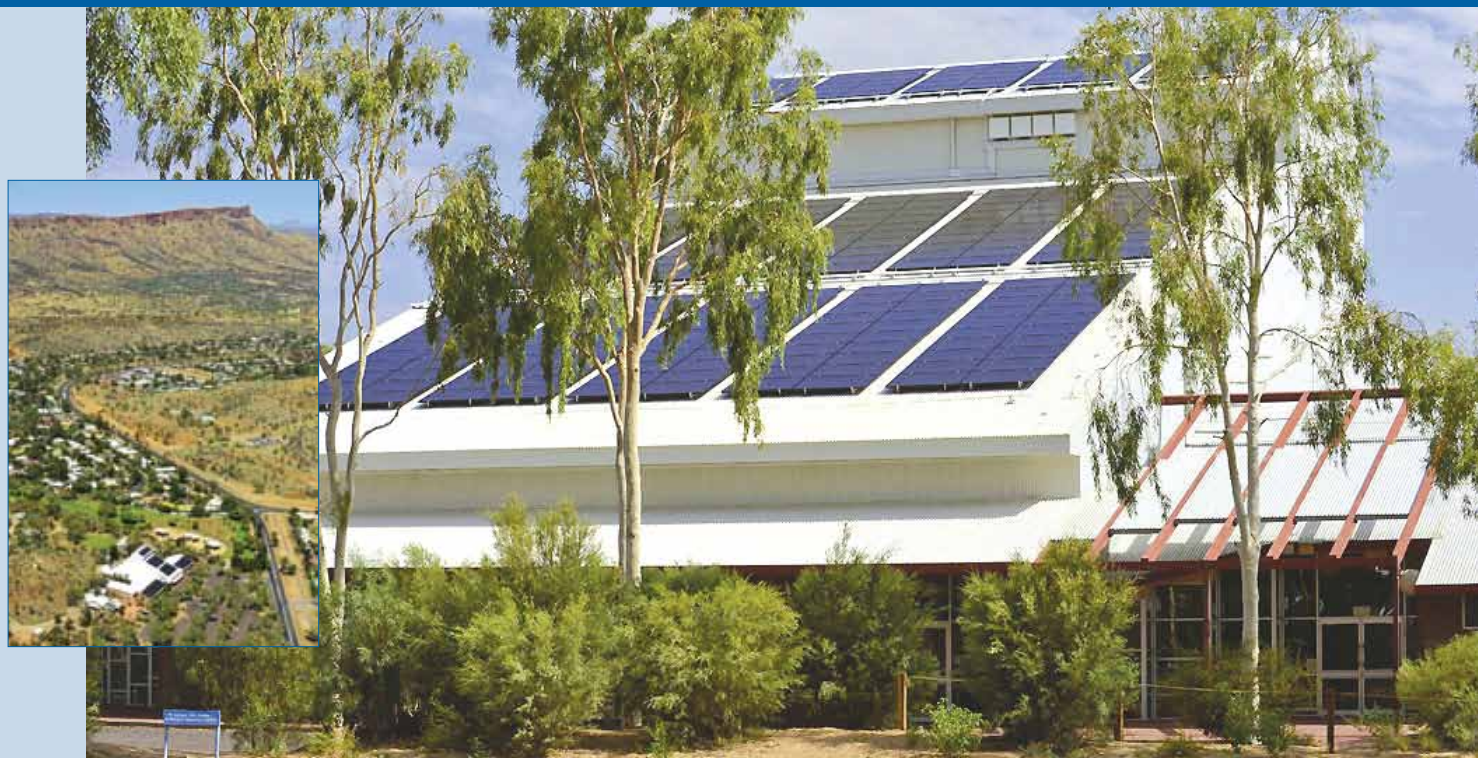
Fig. 1 - Araluen Arts Centre, Alice Springs, 180 kWp solar system using Hanwha Q.Cells QPeak Black modules. Designed by CAT Projects as part of the Alice Solar City and expected to produce 330 MWh per year (Photo: Hanwha Q.Cells).
