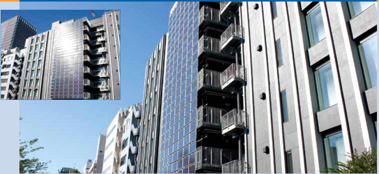
Fig. 3 - Kyobashi OM Building (Chuo-ku, Tokyo), 42 kW, Multicrystalline Silicon PV module.
