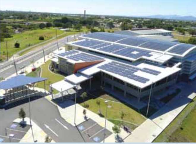
Fig. 2 - The Townsville RSL Stadium 348 kWp PV system for the Townsville Queensland Solar City Project. The system comprises: main curve roof (173 kWp), 2 x flat skillion roofs (155 kWp) and shade structure (20 kWp) using Kyocera KD135 and KD240W modules. The system is expected to generate 510 MWh a year and will provide about half the energy needs of the stadium in winter and around one third of its needs in summer (Photo: Ergon Energy).
