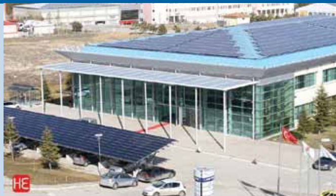
Fig. 2 - 420 kW grid-connected PV system in Ankara, Turkey.
