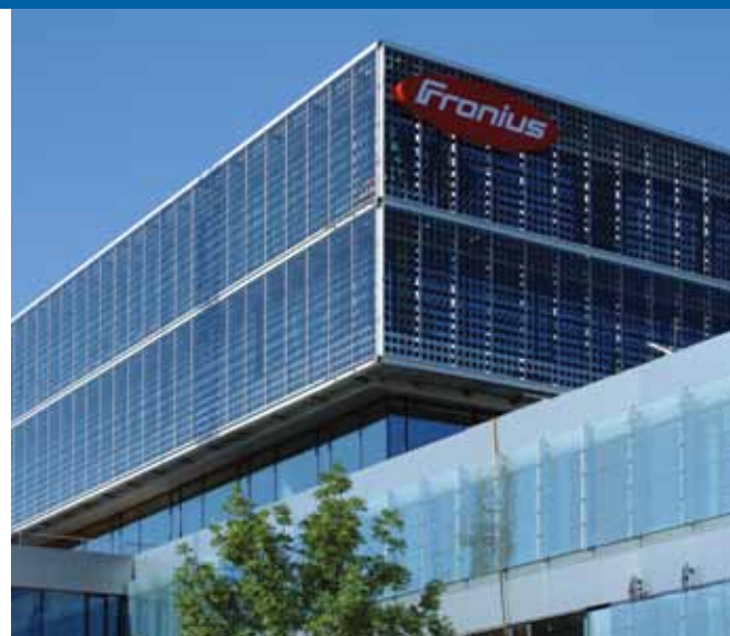
Fig. 1 - PV-glass-glass modules at the Fronius PV inverter factory/Upper Austria (Photo: Ertex-Solartechnik GmbH).
