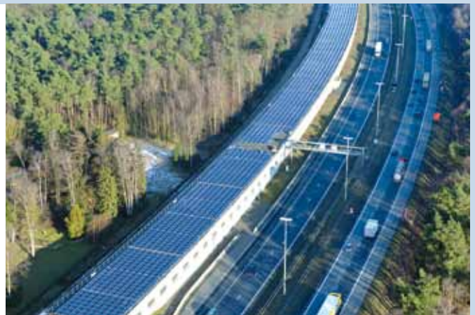
Fig. 5 – Solar Tunnel: The 3,6 kilometer solar tunnel produces enough electricity to power 4 000 trains a year.
