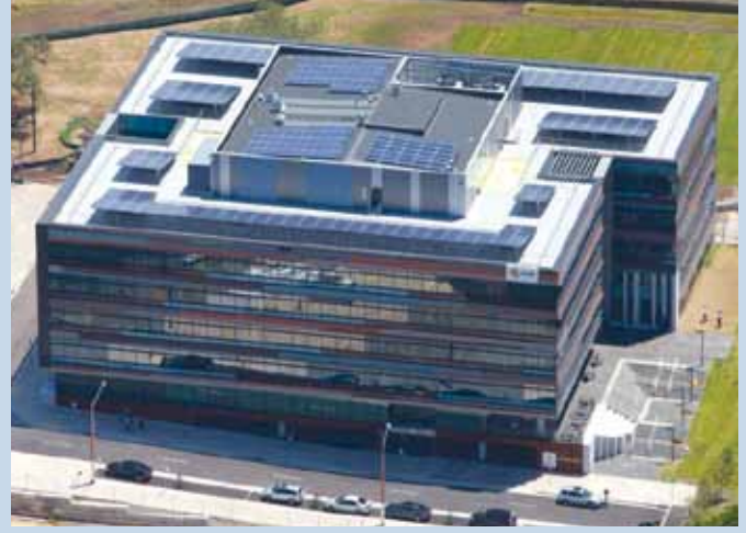
Fig. 3 - 5 Murray Rose Avenue, Olympic Park, Sydney. The 130,5 kWp commercial office rooftop PV system was used to achieve Peak Demand Reduction and Emissions Reduction credits towards a 6 Star Green Star certified office rating. The PV system is also a significant part of the 5 Star NABERS Energy target for building operation (Photo: The GPT Group).
