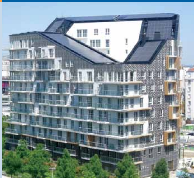
Fig. 1 – Low-energy building in Paris' 17 th arrondissement. 96 kW BIPV designed and installed by Sunvie.
