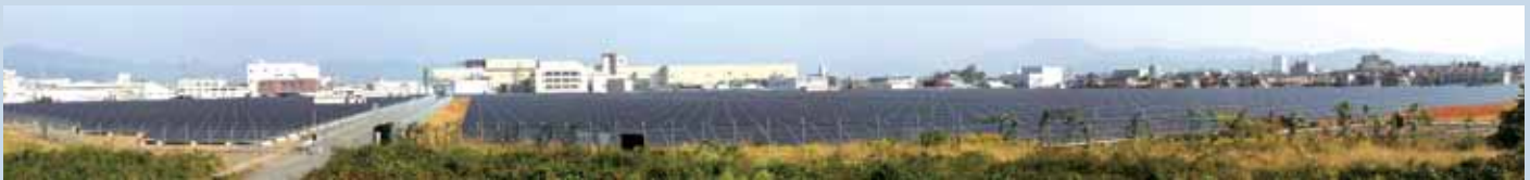
Fig. 2 – SoftBank Kyoto Solar Park (Fushimi-ku, Kyoto City, Kyoto Prefecture), 4,2 MW, Multicrystalline Silicon PV module by Kyocera.
