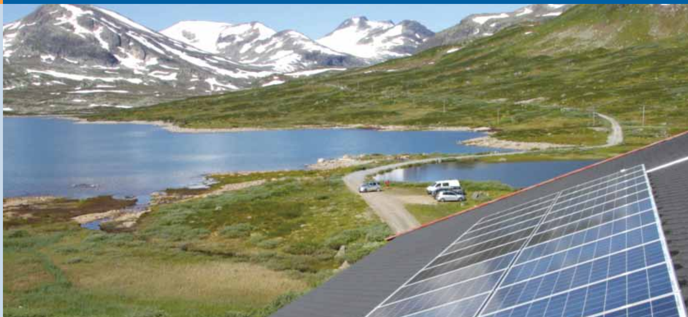
Fig. 2 - PV installation at Tynholmen lodge in the Norwegian mountains. With 22 panels, approx 6 kW, supplied by REC.
