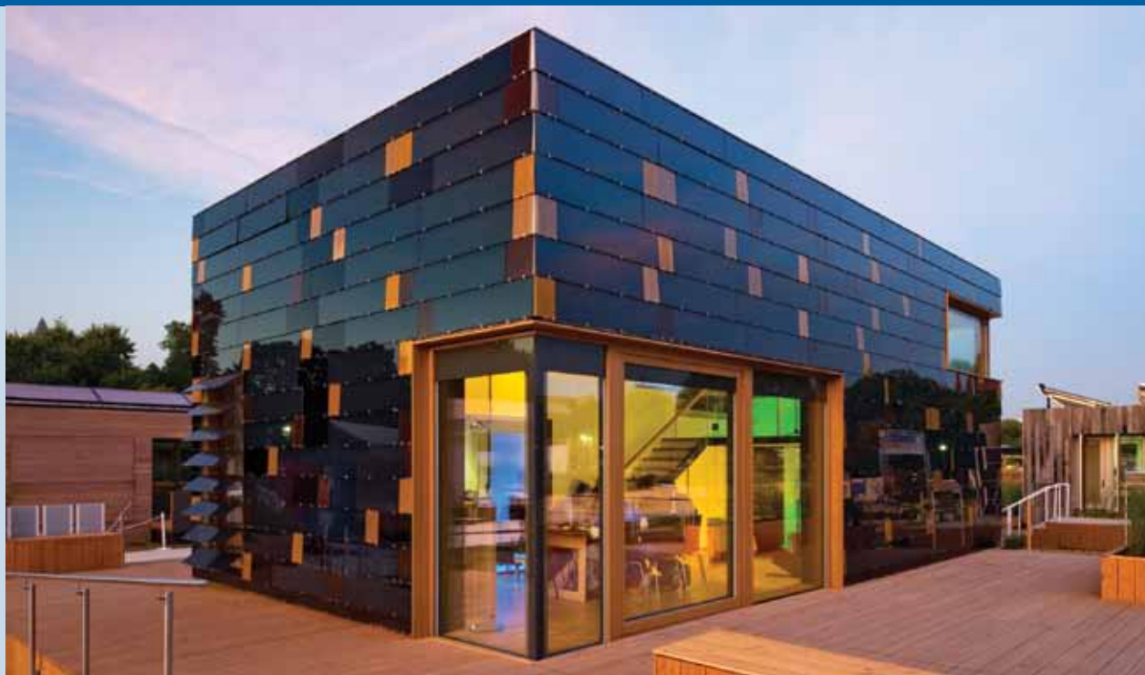
Fig. 1 - Example of a building integrated PV system demonstrating the beneficial combination of CIGS solar modules and modern architecture (Photo: T. Ott).
