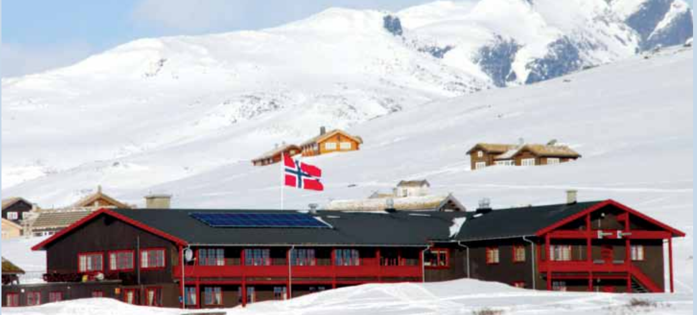
Fig. 1 - PV installation at Tynholmen lodge in the Norwegian mountains. With 22 panels, approx 6 kW, supplied by REC.
