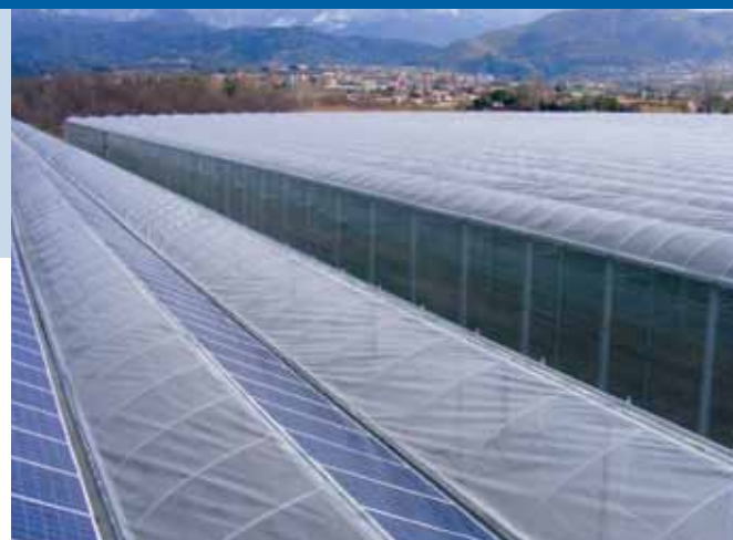
Fig. 3 – 3,0 MW Scaela1 PV Plant on a greenhouse at Cosenza (Photo: Hfv spa)
