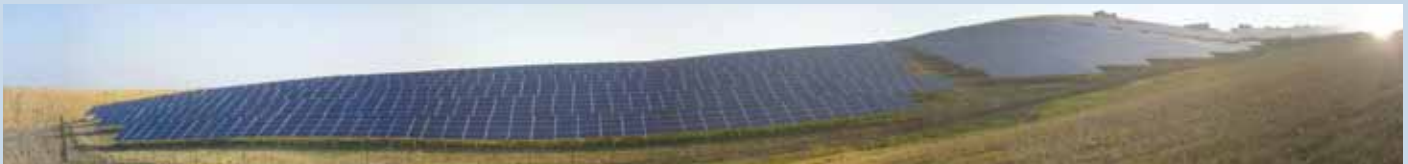
Fig. 2 – 3,5 MW Montenero PV Plant at Campobasso (Photo: Hfv spa).
