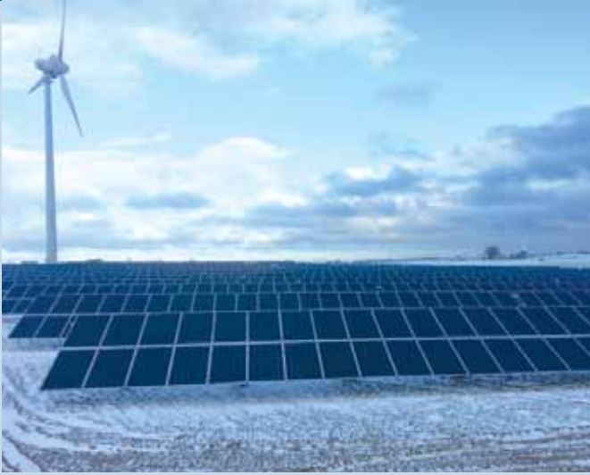
Fig. 1 - In December 2012, the largest PV installation in Sweden to-date, began to operate: 440 kW outside of Simrishamn (Photo: Solect Power).
