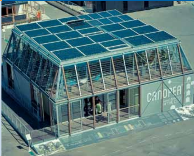
Fig. 2 – Canopea®. Solar-powered housing project designed by Team Rhône-Alpes, winner of the 2012 Solar Decathlon Europe competition. Top of an apartment building with PV/T hybrid collectors.
