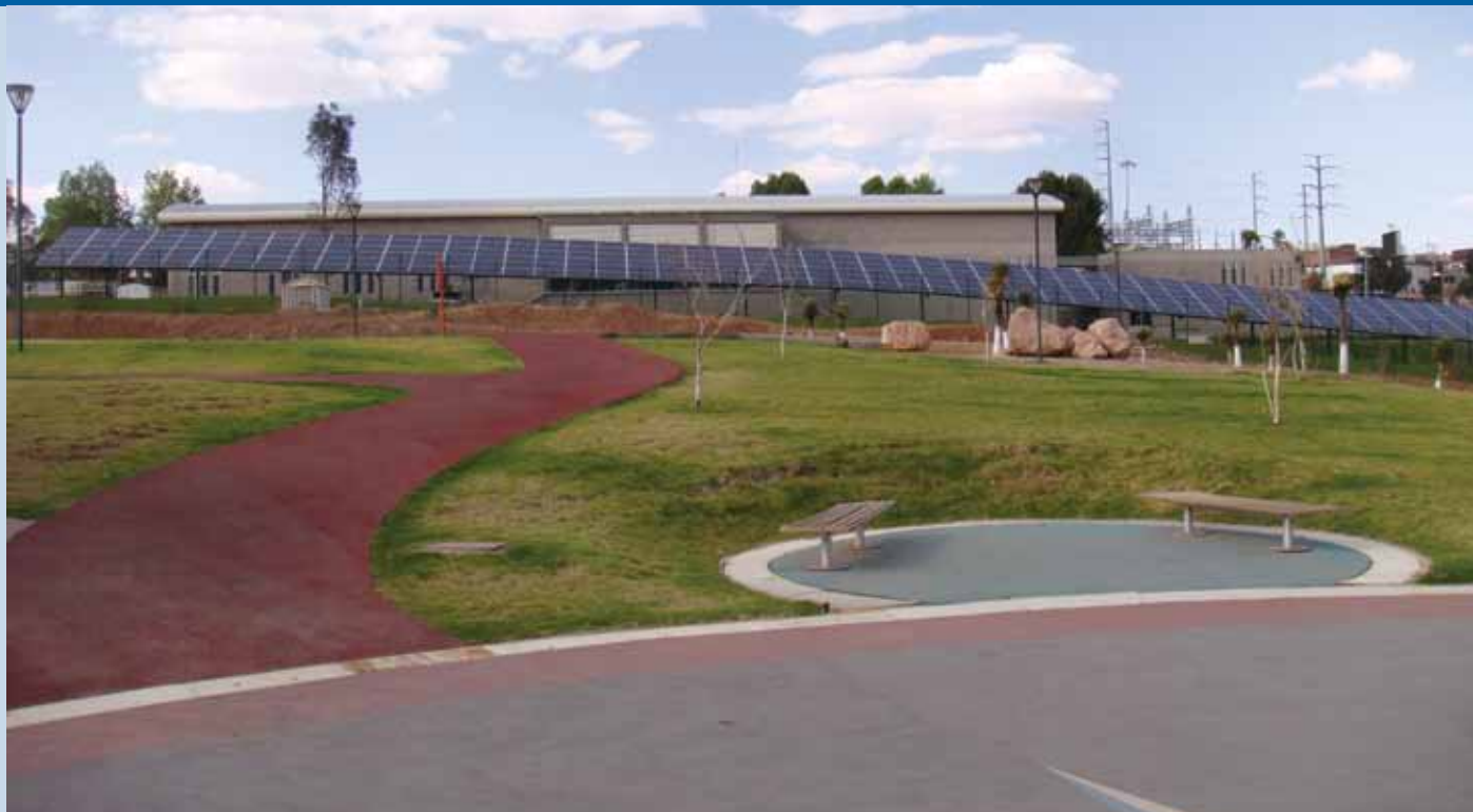
Fig. 1 - 182 kW Grid Connected PV System in Zacatecas, Mexico.
