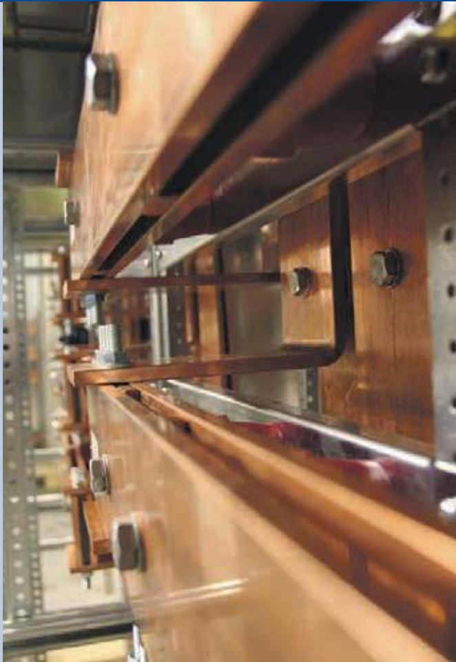
Fig. 1 – Copper busbars.
