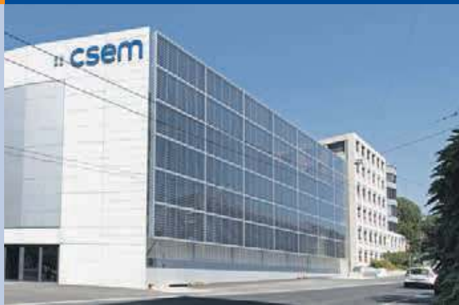
Fig. 4 - New 70 kW PV façade at the CSEM building in Neuchâtel (Photo: CSEM SA).
