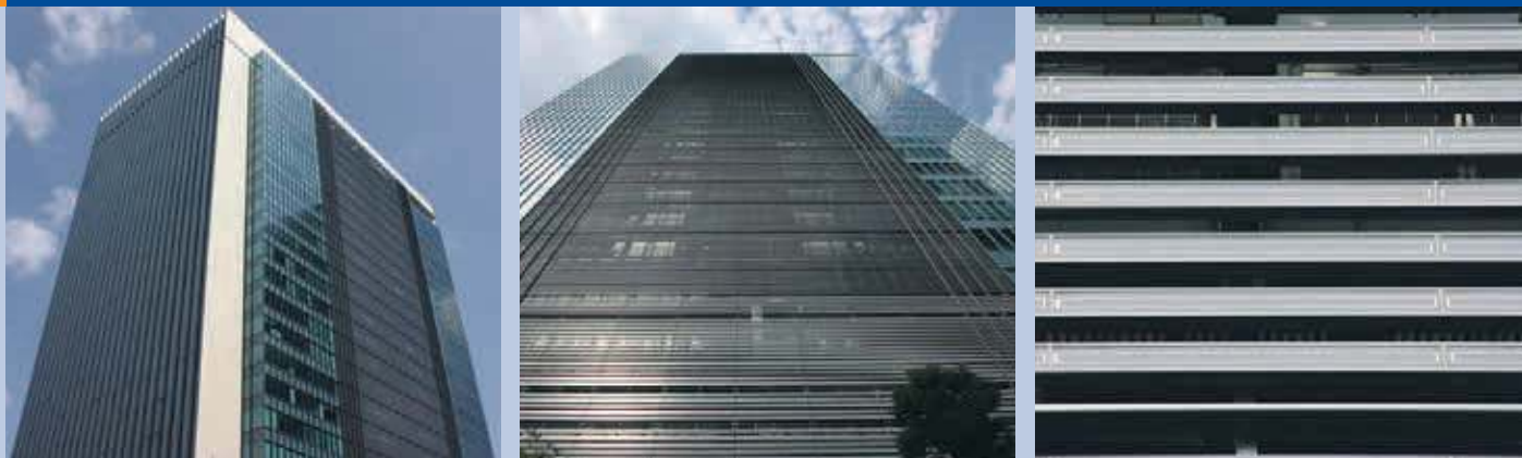
Fig. 2 - Office building "Ochanomizu Sola City" (Chiyoda Ward, Tokyo). Single crystalline silicon PV module: 150 kW.
