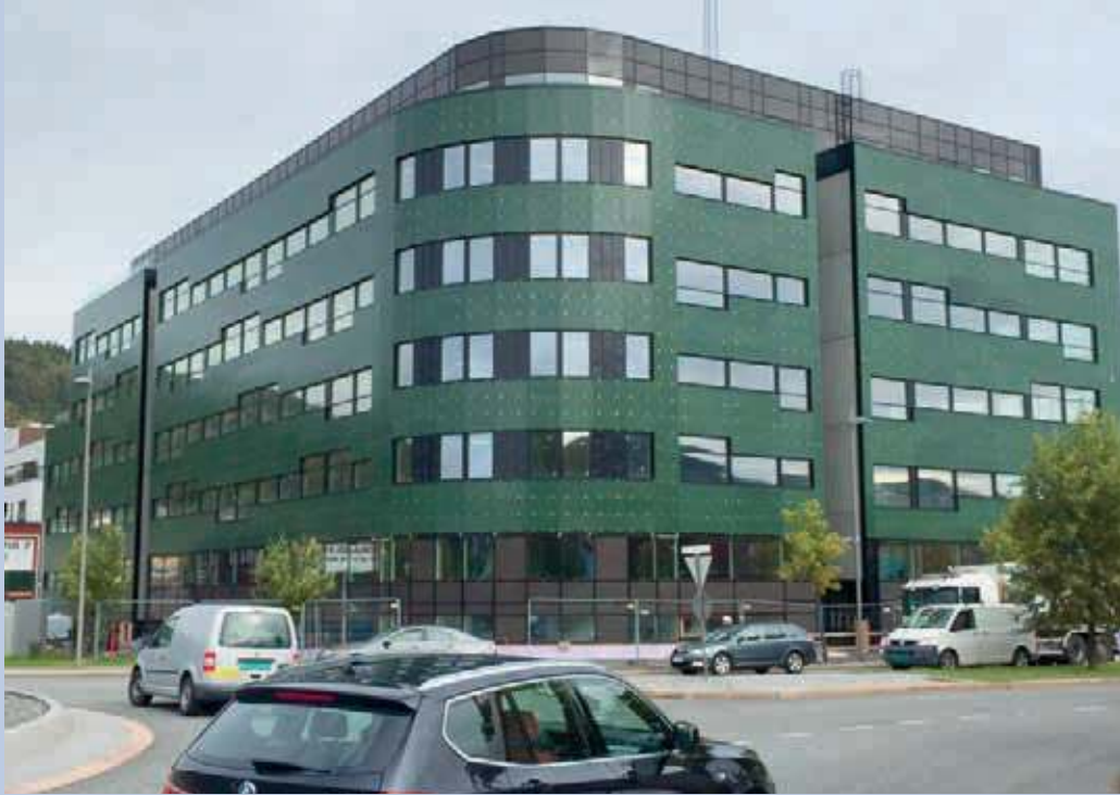
Fig. 1 - 127 kWp of screen-printed glass with integrated PV cells installed in 2015 at Solsmaragden, in Drammen, Norway (Photo: Fusen AS).
