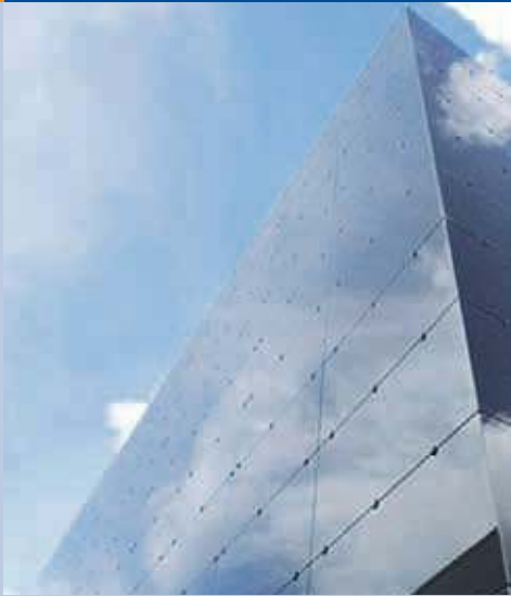
Fig. 3 - BIPV office façade in Spain with a combination of opaque and semi-transparent amorphous silicon photovoltaic glass modules (Photo: © Onyx).
