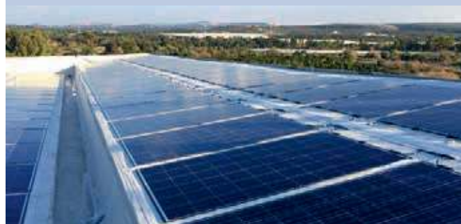
Fig. 2 - Solatics PV Integrated Membrane installation, using the "Direct Attachment" method.
