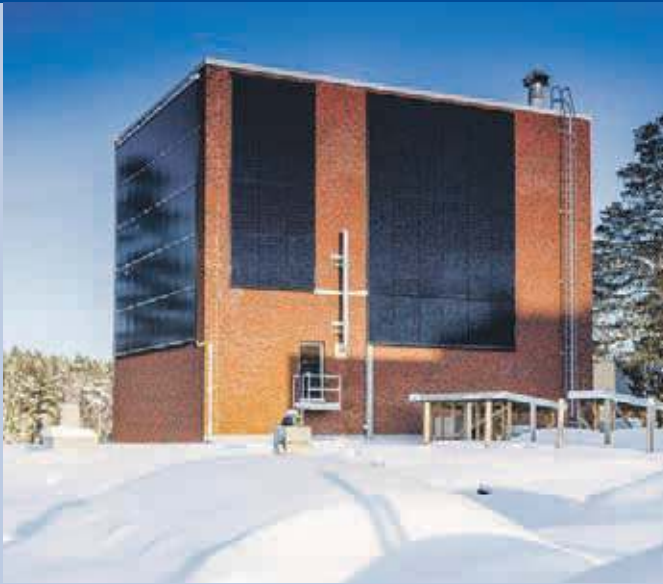
Fig. 1 - Wall-mounted solar PV panels at LUT (Photo: Lappeenranta University of Technology www.lut.fi ).
