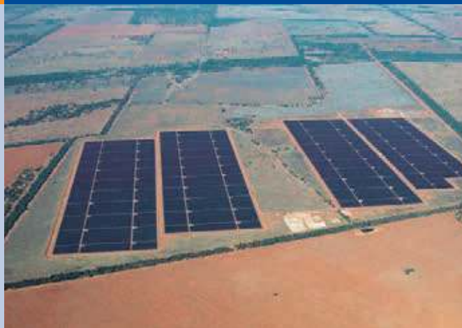
Fig. 2 - The ARENA Solar Flagship Utility Scale Solar Farm, Nyngan NSW. AGL: How we source our energy (Photo: AGL Energy).
