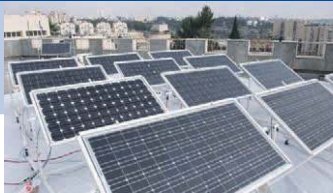
Fig. 1 - First generation BiFacial PV system installed by SolAround, with white background to increase the contribution of the back side of the PV panel. Overall efficiency of SolAround BiFacial panels is expected to be between 25-28 %.
