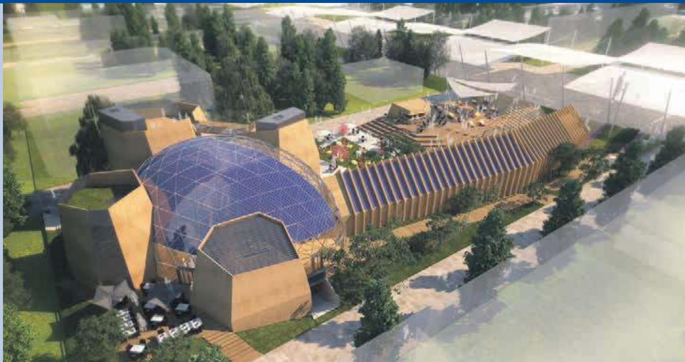
Fig. 1 - The roof of the Belgian pavilion at the Universal Exhibition in Milano was covered with BIPV laminated photovoltaic glass from the AGC Company (either crystalline photovoltaic cells or an organic fill).
