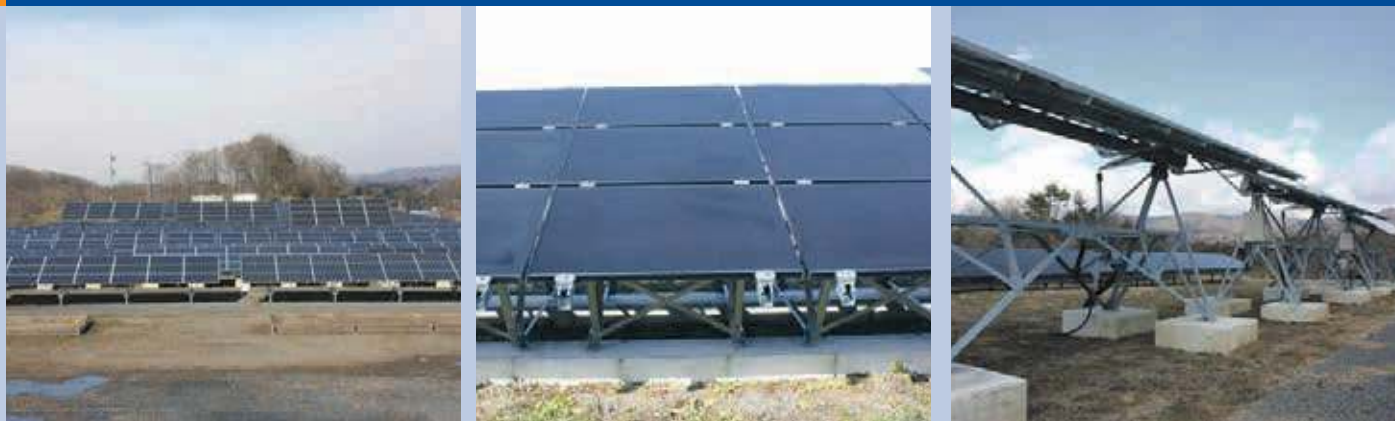
Fig. 3 - Fukushima Airport Mega-Solar Power Plant (Sukagawa City, Fukushima Prefecture, etc.). Total: 1,2 MW (500 kW, 200 kW, 500 kW), 30 types of PV modules including tracking system and various types of mounting structures.
