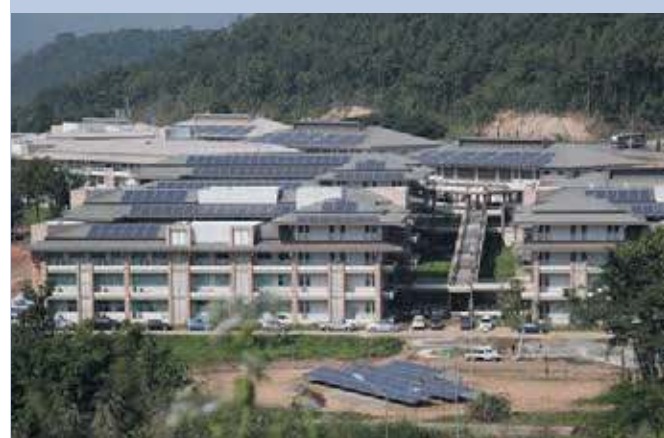
Fig. 2 - 500 kWp PV Rooftop of the Smart Grid System at the University of Phayao (Photos: University of Phayao).
