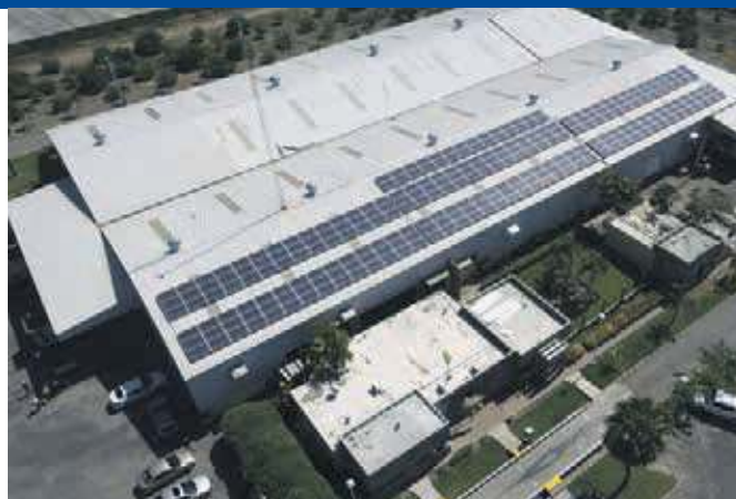
Fig. 1 - 70 kW PV System in a Fruit Packing Plant, Colima MX (Photo: Conermex).
