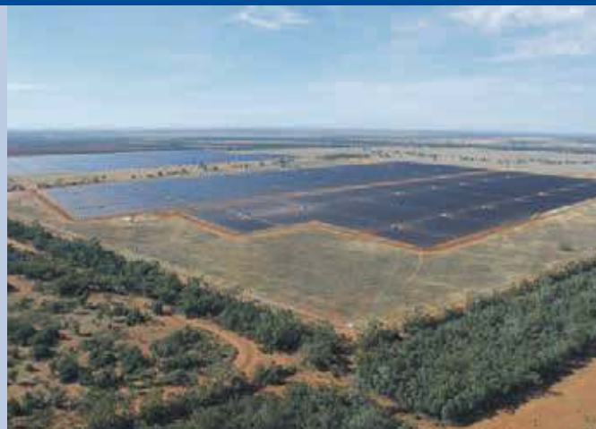
Fig. 3 - The ARENA Solar Flagship Utility Scale Solar Farm, Nyngan NSW (Photo: AGL Energy).
