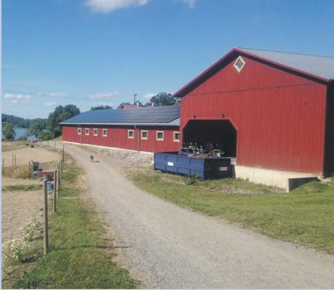
Fig. 1 - 62 kW photovoltaics on barn roof in Bromma Gård, outside of Stockholm (Photo: Solkompaniet).
