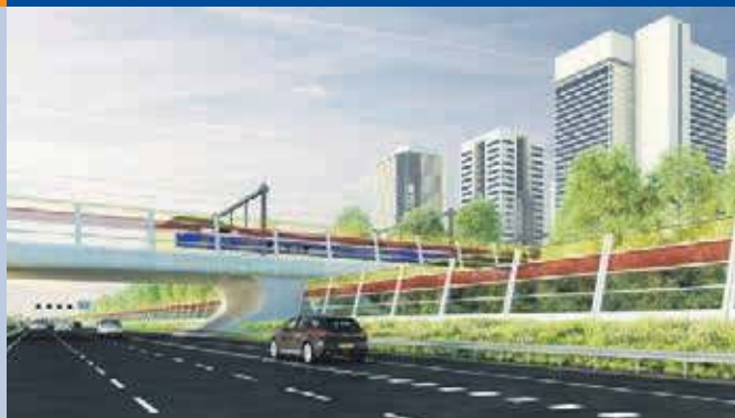
Fig. 4 - Design LSC in solar screen SONOB along highway by Heijmans (Source: Heijmans Bv. http://www.heijmans.nl/nl/solar-noise-barriers-sonob/ ).
