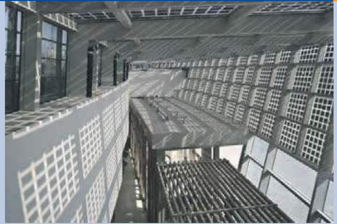
Fig. 4 - Semi-transparent glass photovoltaic modules in the Korean Football Arena entrance lobby.
