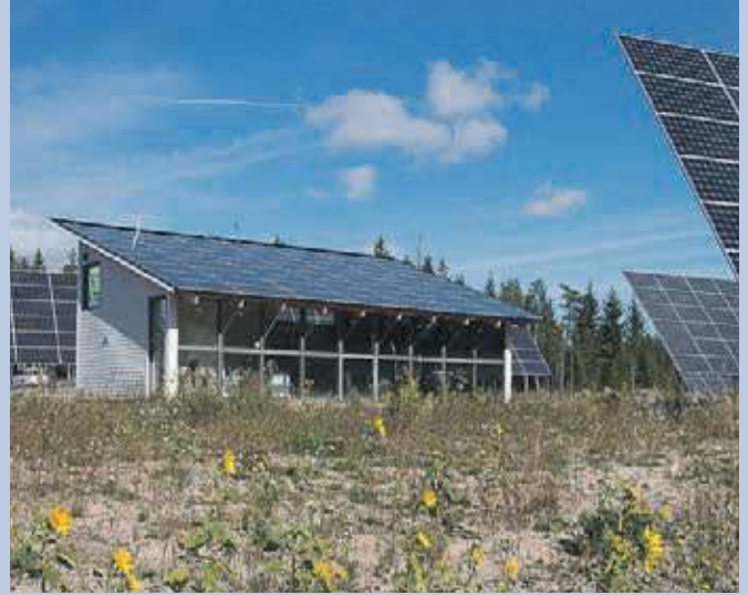
Fig. 2 - Sunflowers and part of the 1 MW PV installation outside of Västerås. A recently published monitoring project has compared the output from fixed, 1-axis and 2-axis tracking systems, with and without power optimizers (Photo: Bengt Stridh).
