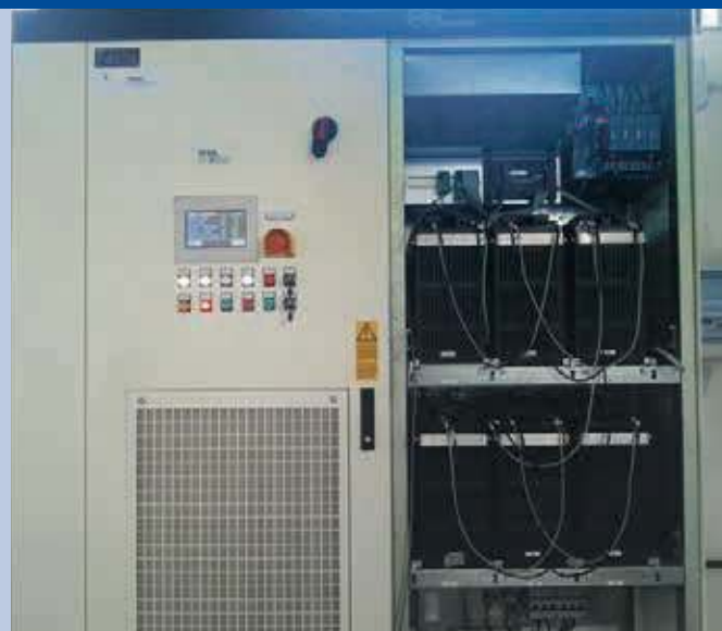
Fig. 3 - Li-Ion Energy storage system (16 kWh) for 14 kWp grid connected PV plant on Lampedusa island (Photo: ENEA, www.enea.it ).
