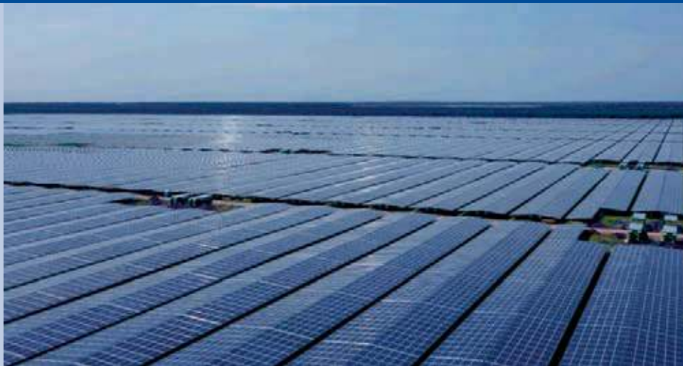
Fig. 3 – 230 MW PV plant, near Bordeaux, mounted on fixed structures with an east-west orientation (Photo: Neoen, Clemessy).
