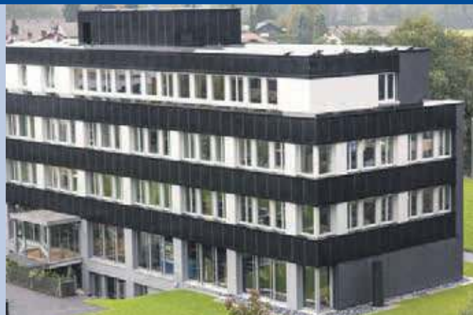
Fig. 5 - PV rooftop and façade systems on an office building in Flums (Photo: © NET Ltd. / DanielForster.com).
