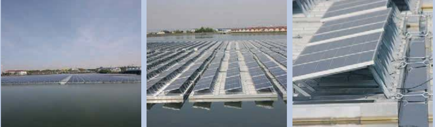
Fig. 1 - Floating PV Power Plant (INFINI Hyogo Daikyu Power Plant) (Inami Town, Hyogo Prefecture). Multicrystalline silicon PV module: 250 W x 6 846 modules (by INFINI) 1,7 MW.
