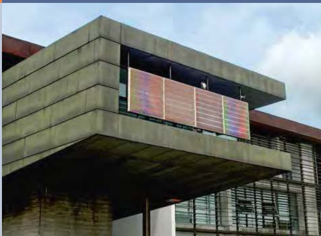
Fig. 4 – Demonstrator installed in ITMA building out of BIPV elements (transparent PV and LED integrated) developed in the ETFE-MFM project.
