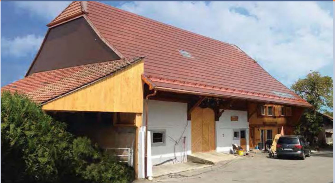
Fig. 2 - A southwest view of the PV installation on a farm house in Ecuivillens, Fribourg, Switzerland. With their terracotta appearance, these innovative PV roof tiles provide a perfect integration into the townscape (photos: © CSEM & © ISSOL).
