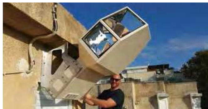
Fig. 2 - Solight installing its lighting system.
