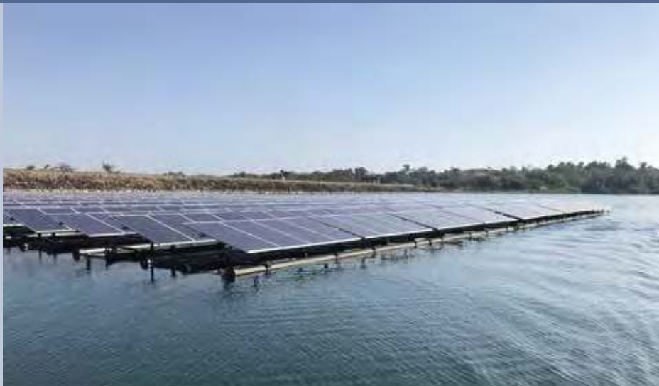
Fig. 2 - 250 kW Solar Floating Project by EGAT at Sirinthorn Dam, Ubon Ratchathani Province. This is a project for preparation and development of Solar Floating Systems in Thailand with the goal of continuing to target GW in 2021 (Photo: EGAT).
