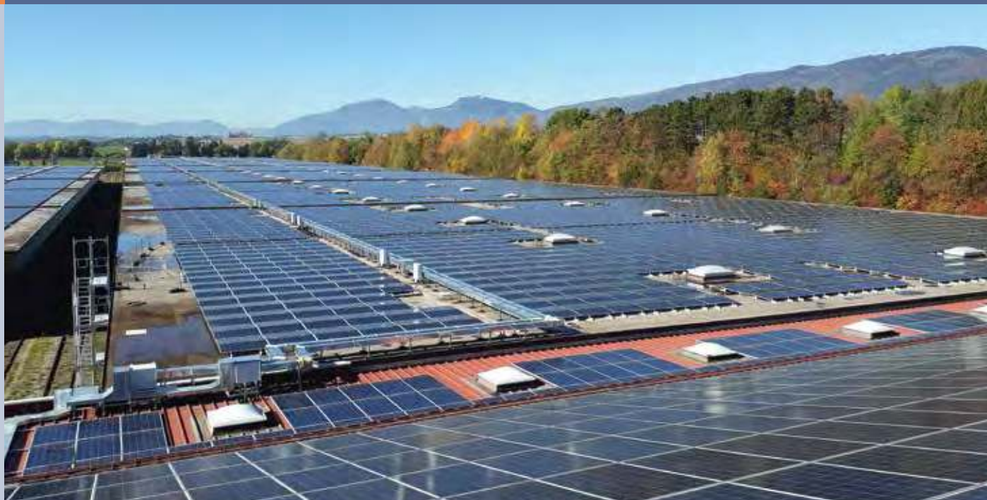
Fig. 3 - PV System at Philip Morris in Onnens, Switzerland. The entire system (mounted on several roofs) is presently the largest PV installation in Switzerland; with a capacity of 8,3 MWp, it produces approximately 8 GWh of solar power per year (Photo: © aventron AG).
