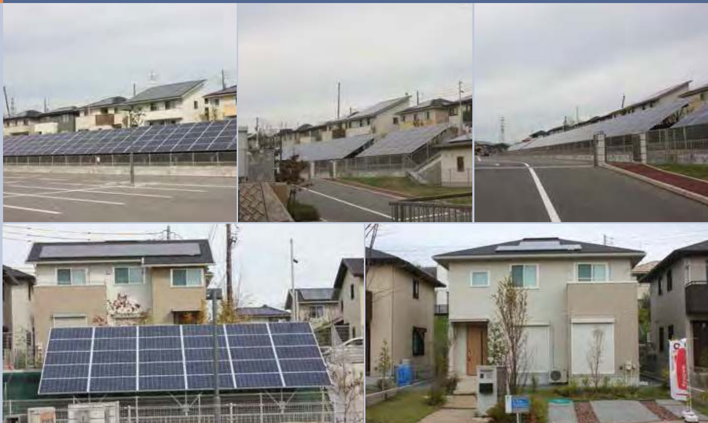
Fig. 2 - Smart Town with PV systems installed on all houses as standard (Sma x Eco Town Hidamari no Oka) (Kuwana City, Mie Prefecture). Houses: 66 residential PV systems (ca. 330 kW in total), Ground-mounted PV system: 100 kW, Multicrystalline silicon PV modules (by Sharp).
