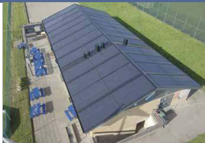
Fig. 1 - PV/T Energy Day at Stenløse Football Club: The innovative "Hercules energy roof" with efficiency exceeding 50 %, was developed and produced by RACELL A/S for the Stenløse club building. The old worn-out and leaking roof was replaced by the new water-tight solar roof. The 7,5 m 2 self-bearing light-weight Hercules modules were fixed directly on-top of the wooden battens, thus the installation took 2 days only. The hybrid PVT roof has a capacity of 520 W/m 2 (electricity 180 W p /m 2 and heat energy 340 W p /m 2 ). The total south roof area is 180 m 2 . The project was supported by the Danish Energy Agency EUDP (Photo: RACELL).
