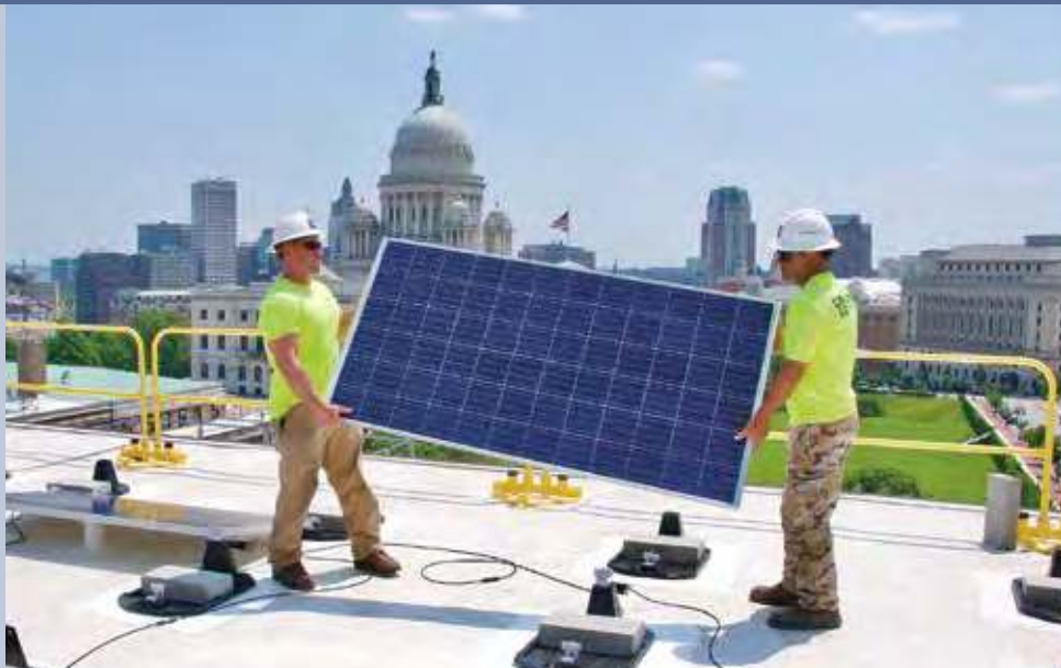
Fig. 2 - Phil Doucette (left) and Jim Mitchell (right) of Newport Renewables install solar panels on the Powers Building, part of a 330 000 kWh, 890 panel project covering three government buildings in the Capitol Hill complex. The Rhode Island Statehouse is visible in the background (Photo: Robert Beadle).
