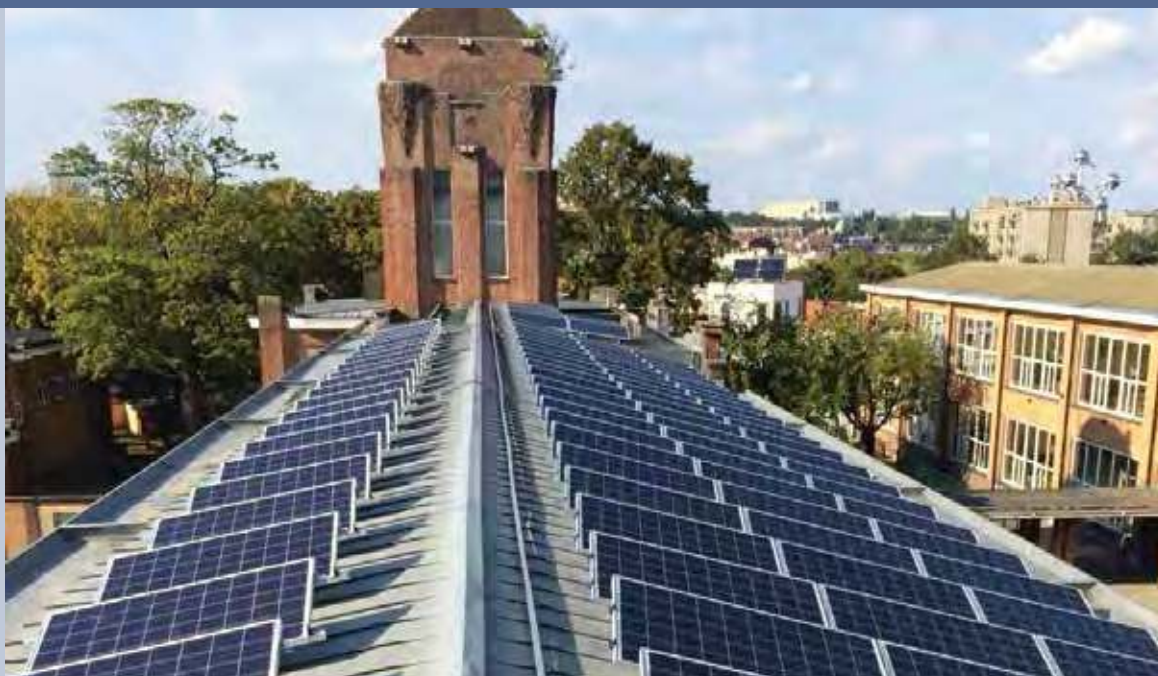
Fig. 2 - Energiris PV project in Brussels: Cooperatives are increasingly active to allow schools or other public buildings to install PV on their roofs and citizens to invest in projects.
