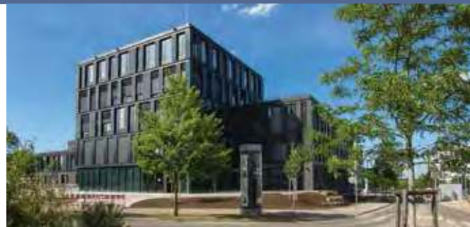
Fig. 1 - CIGS thin film solar façade system (Photo: © ZSW Stuttgart / www.zsw-bw.de ).
