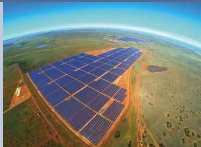
Fig. 5 – 75 MW PV plant built by COBRA in Kimberley, Rep. of South Africa (Photo: ©Grupo Cobra).
