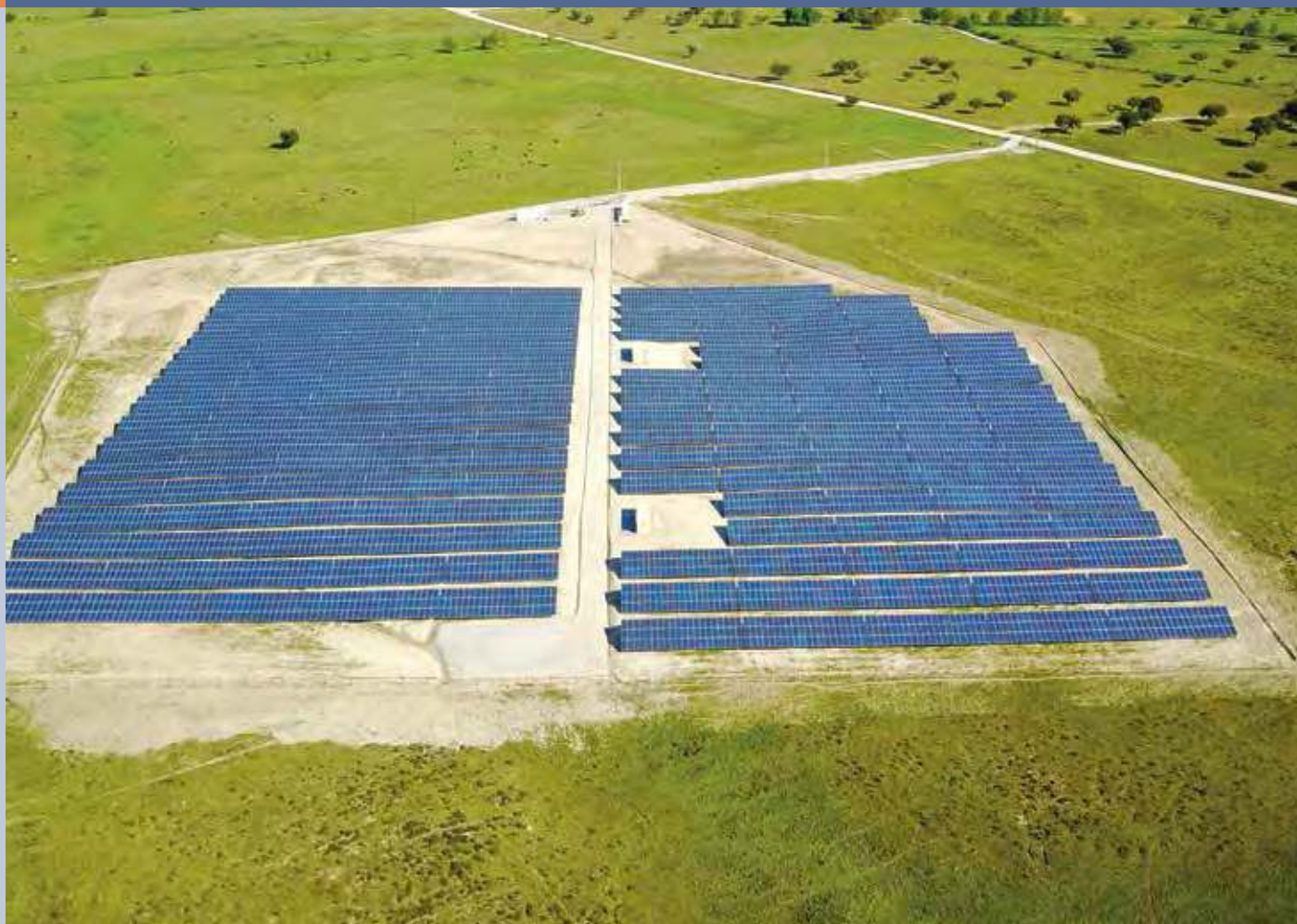
Fig. 2 - 2,5 MW PV Power Plant at Monte das Flores (Photo: APREN).
