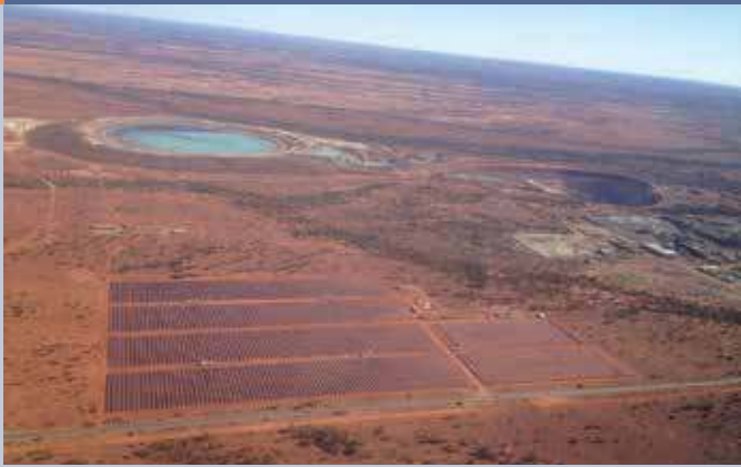
Fig. 3 - The DeGrussa Solar Farm. The DeGrussa Solar Project was successfully commissioned at Sandfire's DeGrussa Copper-Gold Mine. It has 34 080 solar PV panels with a single-axis tracking system mounted on 4 700 steel posts.
