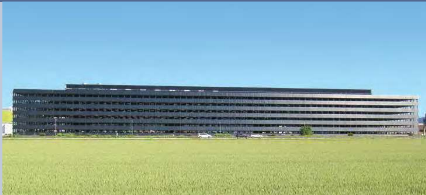
Fig. 1 - Swissolar Prize Winner 2017: The most powerful PV façade in Switzerland on the F. Hoffmann-La Roche AG's parking garage in Kaiseraugst, Switzerland. This façade system has a total installed capacity of 633 kWp and an estimated production of 473 000 kWh per year (Photo: © BE Netz AG, Ebikon).
