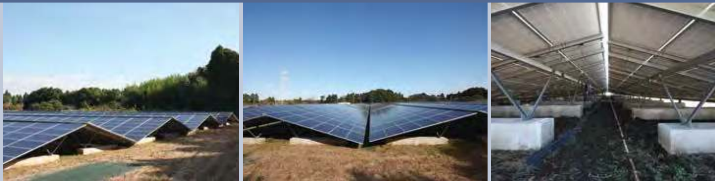
Fig. 1 - Ground-mounted PV System arranged in the east-west direction with an M shape (F Nagara PV Power Plant) (Nagara-machi, Chosei-gun, Chiba Prefecture). 1,905. 1 kW Multicrystalline silicon PV module (by Suntech) (315 W).
