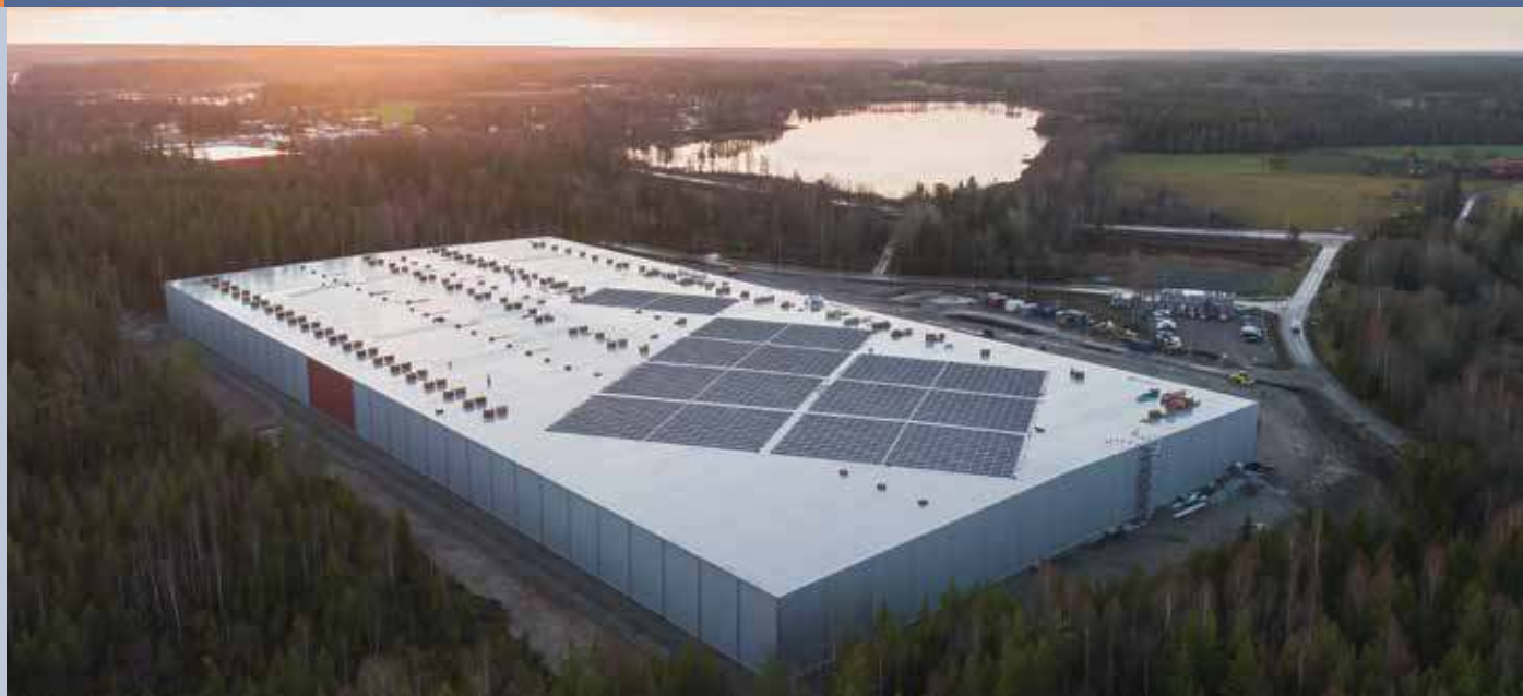
Fig. 2 - Apotea's warehouse and logistic center in Morgongåva - 1 500 kW - Sweden's largest roof-mounted PV system (under installation) (Photo: Gustaf Kumlin / Apotea.se).
