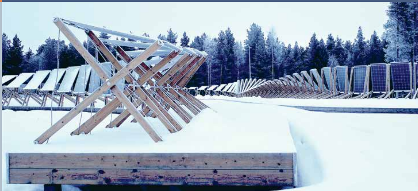
Fig. 2 - Solvåg – Piteå – 117 double-sided solar panels from Prism Solar (USA) – 36 kWp – Yearly production 45 MWh (Photo: Warm in the Winter The facility is both a research project and an open green park and social meeting place. It contains 117 double sided solar panels that capture sunlight on the front and reflect light on the back. These are located against different point of the compass and with different angles of inclination towards the sun).
