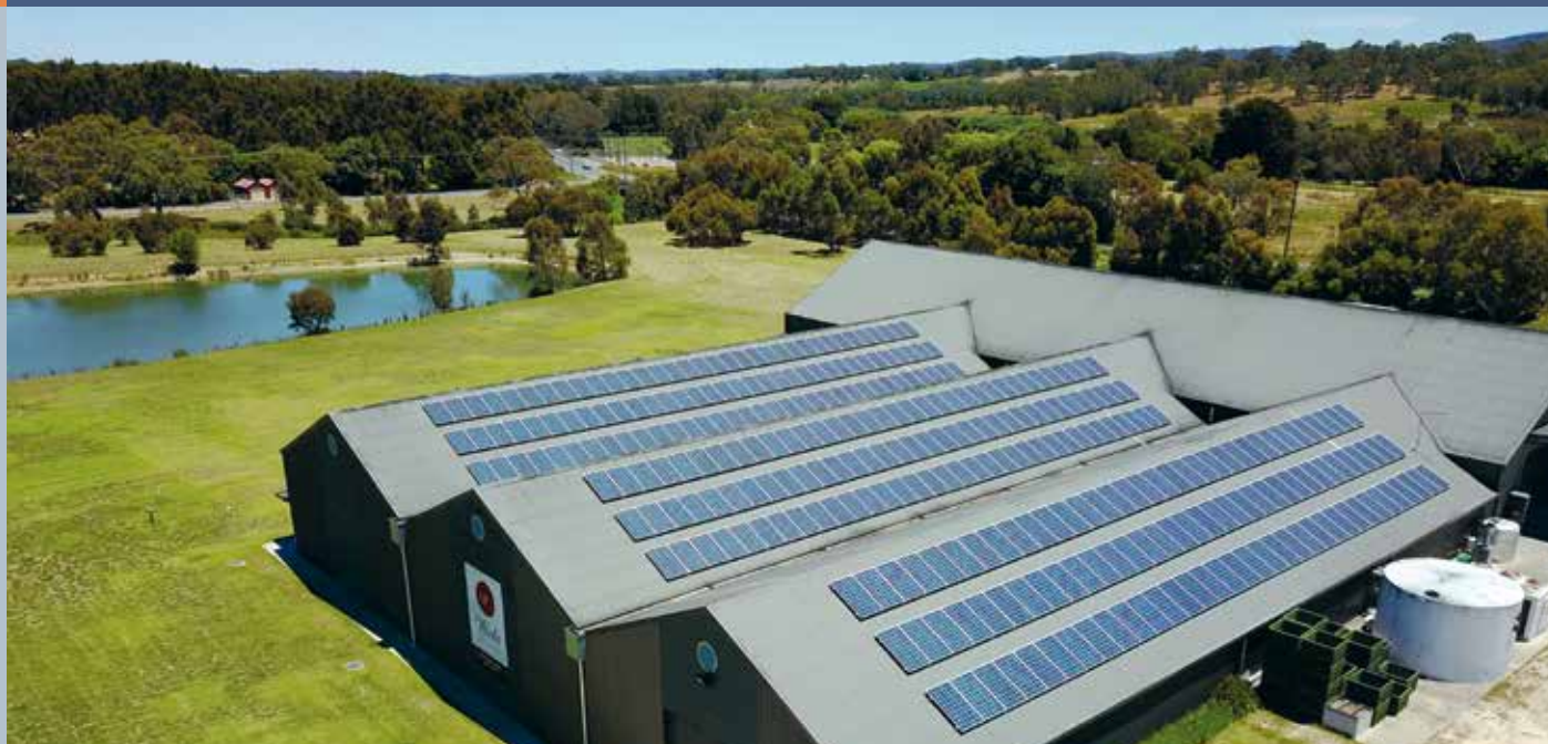
Fig. 3 - Wicks Winery Estate, Woodside, South Australia. Sold and Installed by Venergy Australia (Photo: Matt Wilkins, Venergy Australia).
