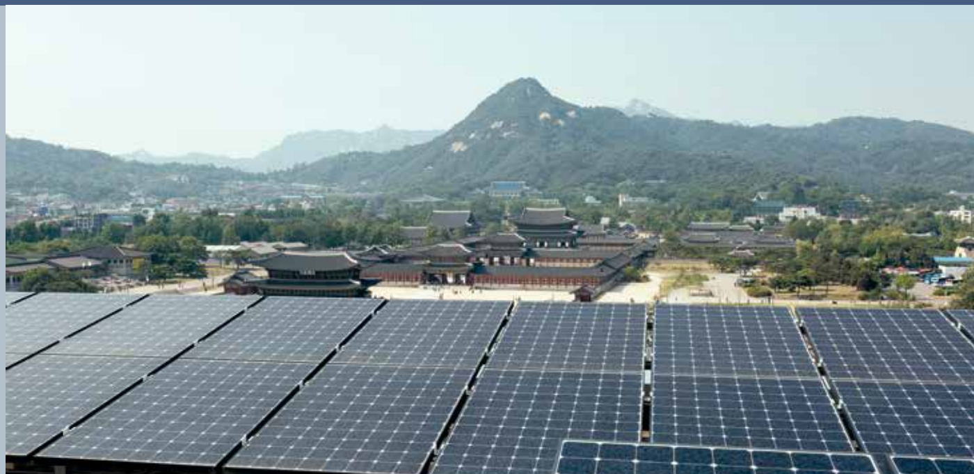
Fig. 1 - Roof mounted PV system at National Museum of Korean Contemporary History, Seoul, Korea.
