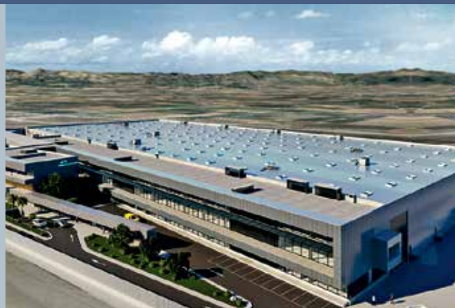
Fig. 5 - New Power Electronics factory in Valencia.
