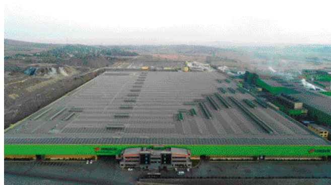
Fig. 1 - One of the largest rooftop PV power systems consisting of thin-film PV modules in Osmaniye (10 MW) [21].
