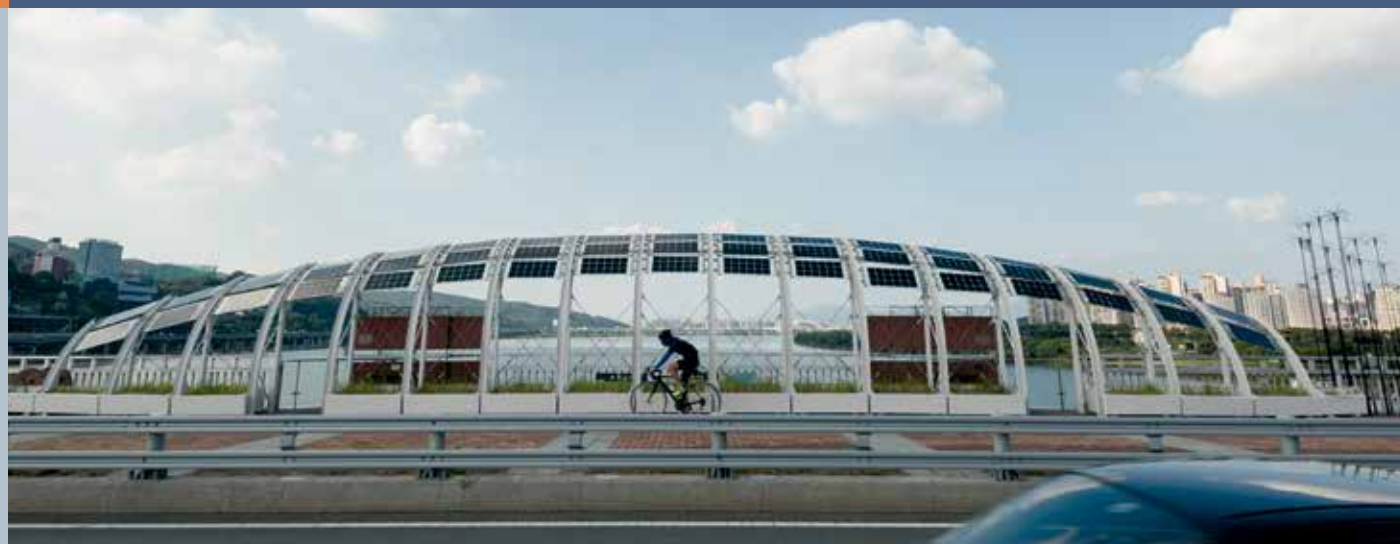
Fig. 3 - Gwangjin Bridge, Seoul, Korea.
