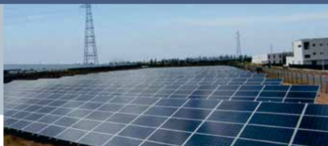
Fig. 2 - 2 MW power plant of the Atlantic Industrial Free Zone of Kenitra.
