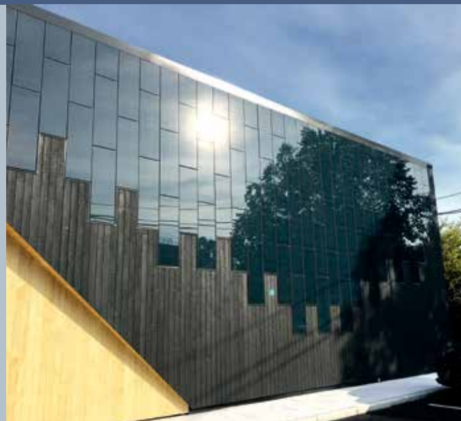
Fig. 2 - Wall of a supermarket in the Oslo area, where the façade is a combination of building integrated PV panels and wood materials. This project also received support from ENOVA SF. In addition to combining energy efficient technologies, this project made extensive use of wood materials in the building design (Photo: Trygve Mongstad, Solenergi FUSen AS).
