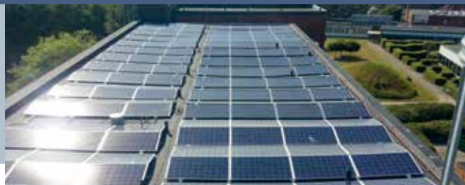
Fig. 2 - Roof top system from the hospital in the city Skive. The power of the system is 61 kWp. System delivered by Helge Andersen, Solarpark DK A/S, Denmark.
