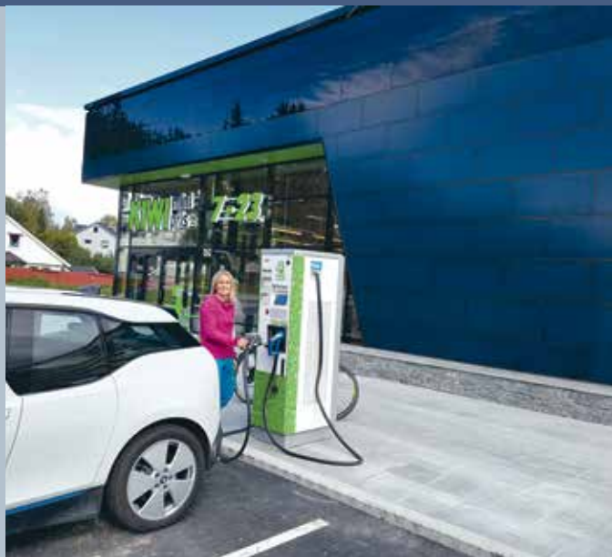
Fig. 1 - This supermarket in Trondheim has a combination of building integrated PV panels in the façade, standard solar panels on the roof, battery storage, and energy wells. The project received support from ENOVA SF due to its innovative combination of energy efficient technologies (Photo: Geir Fikke, Solenergi FUSen AS).
