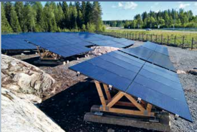
Fig. 1 - Solar PV ground installation at Mikkeli, Finland (Photo: Etelä-Savon Energia Oy; Heidi Mikkonen).
