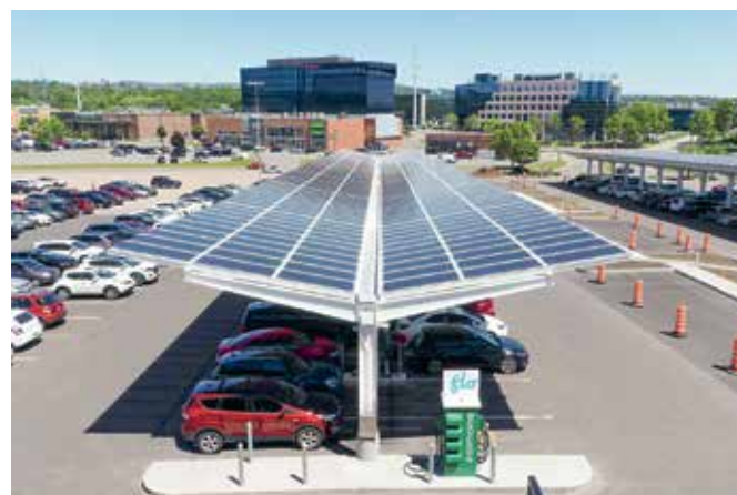
Fig. 1 - Simons department store 1,060 MW PV system located in Québec City is Québec's largest PV system.
