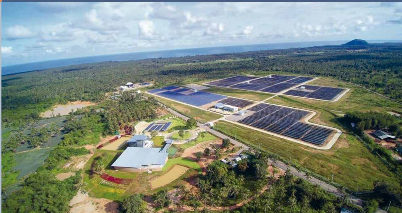
Fig. 2 - 5 MW Tap Sa Kae Solar Power Plant operated by EGAT combines 4 different solar PV technologies. The plant was integrated with learning and research center in the field of solar PV efficiency, energy-efficient building design, and edutainment center that welcome students and interested person to visit and immerse themselves in renewable energy in the Lower Central Region of Thailand.
