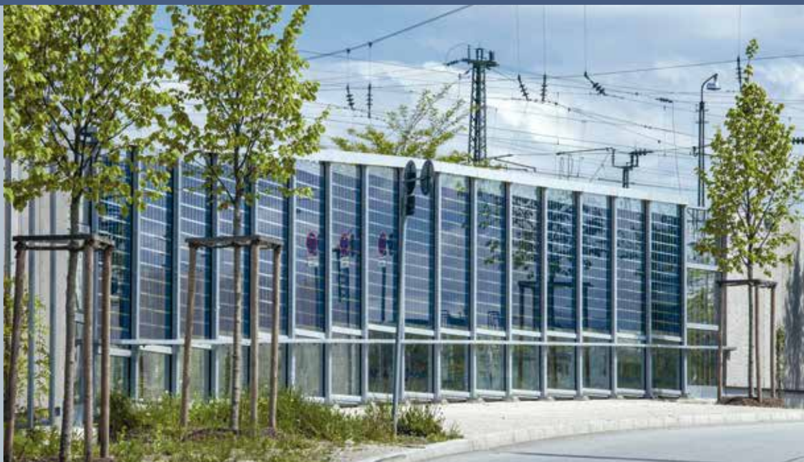
Fig. 1 - PV integrated sound protection wall (Photo: © BMWi / Maria Parusell).
