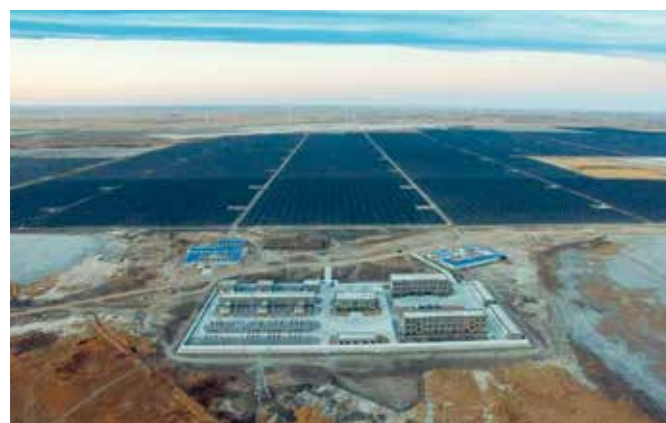
Fig. 2 - Top Runner Project, Baicheng (Photo: PVmen).
