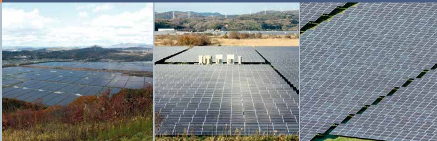
Fig. 3 - Ground-mounted PV System (Setouchi Kirei PV Power Plant) (Setouchi City, Okayama Prefecture). Approximately 235 MW multicrystalline silicon PV modules "TSM-260PC05A" (by Trina Solar) and PV modules (by Yingli Green Energy).
