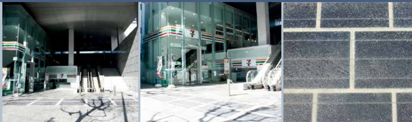
Fig. 1 - Road Surface PV System (Seven-Eleven Chiyoda Nibancho Store) (Chiyoda Ward, Tokyo). About 10,000 kWh/year for the installation of 100 m 2 .
