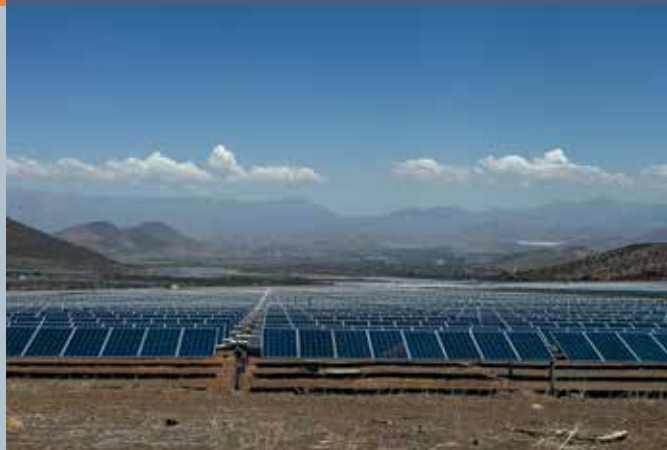
Fig. 4 - Quilapilun Solar PV plant 40 kilometers north of Santiago, 110 MWp operated by EDF Energies Nouvelles.
