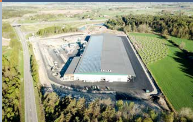
Fig. 3 - Derome Plusshus's warehouse and logistic center in Varberg - 600 kWp. (Photo: Derome Plusshus).
