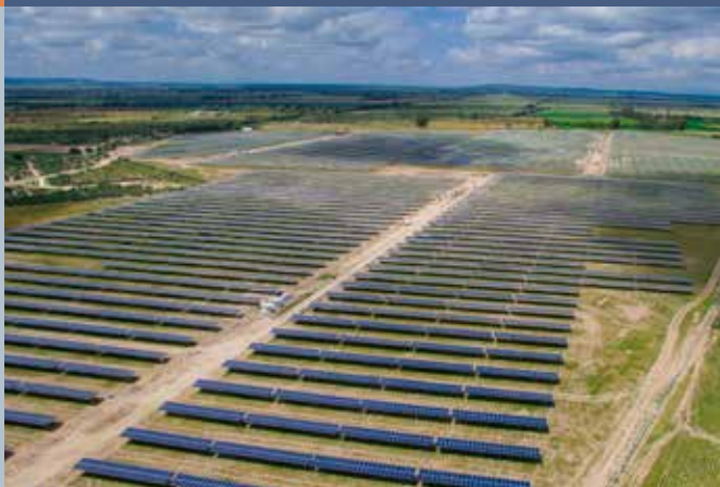
Fig. 4 - PV plant under construction with Soltec's horizontal 1-axis PV trackers.
