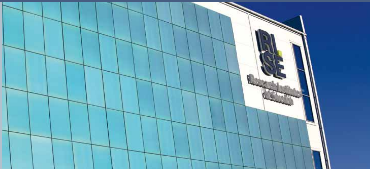
Fig.1 - RISE - RISE EMC-lab "Awitar" in Borås - 82 kWp - Yearly production 48 MWh (Photo: Anna Åberg, Welcome eventbyrå).
