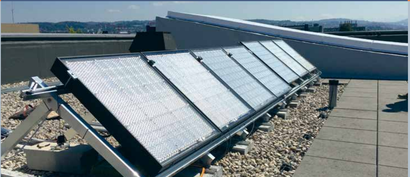
Fig. 3 - High efficiency pilot PV system by Insolight which uses a unique module design: The panel's protective glass embeds a grid of lenses which concentrate the direct sunlight on an underneath array of high-performance space-grade solar cells. An integrated tracking system keeps each cell in focus regardless of the sun's position without active tracking of the modules. Efficiencies of 29 % have been demonstrated (Photo: © Insolight).
