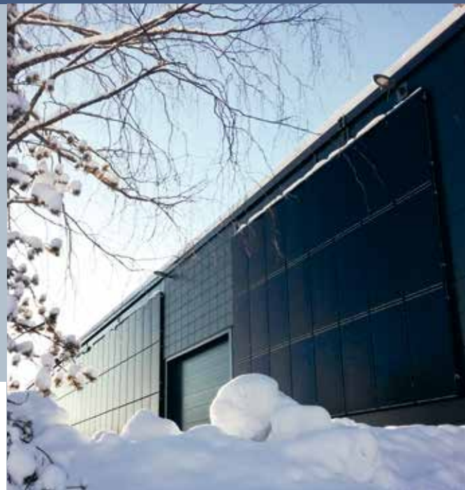
Fig. 2 - LUT University solar PV wall installation in Lappeenranta, Finland (Photo: Jero Ahola).
