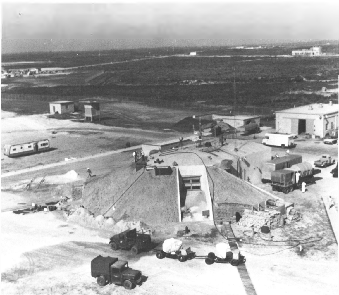
Blockhouse used by Project Vanguard at Cape Canaveral. The horizon window overlooks the launch pad.
