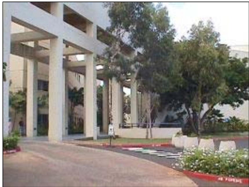
Wilcox Memorial Hospital, Lihue
