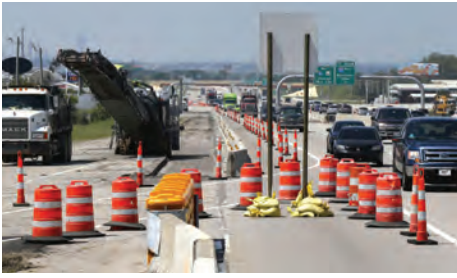
Tulsa often leverages money from the Department of Transportation to help fund stormwater improvements to its road infrastructure.
