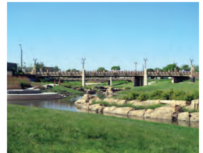
Lincoln's flood mitigation projects were part of a larger community redevelopment project, which included Union Plaza Park.
