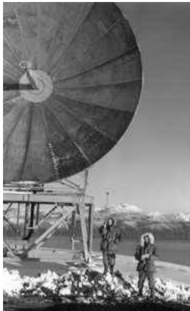
Fig. 5-21. Bell Labs designed the DEW (Distant Early Warning) system Line of radar installations to detect enemy bombers. The DEW Line was stationed across the artic of Canada. [1956 photo courtesy of Alcatel-Lucent USA Inc. / Bell Labs.]
