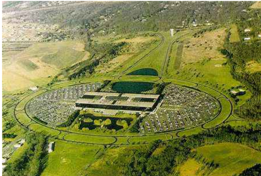
Fig. 4-1. Aerial photo of the Holmdel building, originally designed by Eero Saarinen, and the parking lots, roads, and ponds. The building was expanded in 1984. [Courtesy of the AT&T Archives and History Center.]
