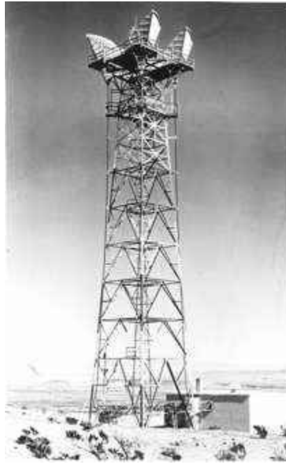
Fig. 5-12. Long-distance telephony utilized a series of microwave towers about every 26 miles to relay signals across the United States. The horn antenna, invented at Bell Labs, allowed radio waves to be polarized and doubled the capacity of earlier systems. [1962 photo courtesy of Alcatel-Lucent USA Inc. / Bell Labs.]
