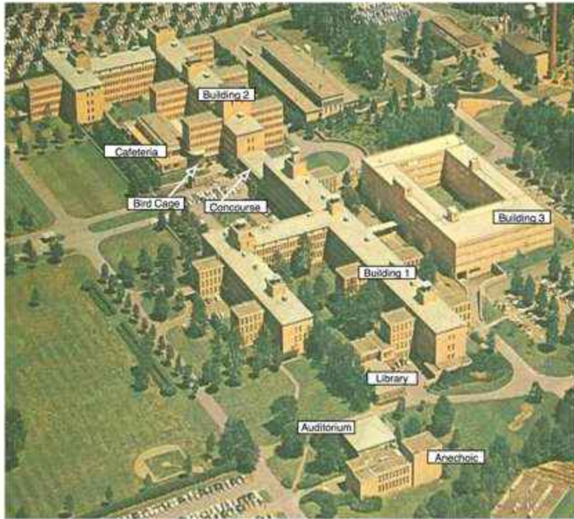
Fig. 2-1. Aerial photograph of the Murray Hill, New Jersey facility on Mountain Avenue in the mid 1960s. Research and development were performed in Building 1 (completed in 1941) and Building 2. A Concourse connected Buildings 1 and 2 on their second floors. A glass-enclosed circular staircase (called "the bird cage") went from the second floor to the Cafeteria on the ground floor. The computer center, medical offices, patent department, and administration were in Building 3 (completed in 1959). The Library was at the western end of Building 2 on the ground floor. The Auditorium and Anechoic Chamber were separate buildings on the western end of the property. [Photo courtesy of Alcatel-Lucent USA Inc. / Bell Labs. Captions by A. Michael Noll.]
