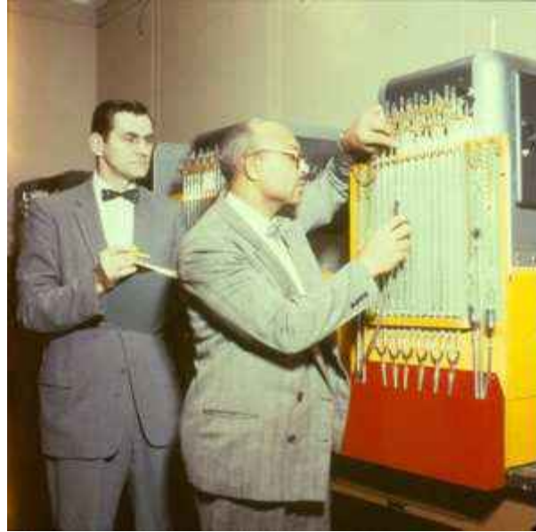
Fig. 9-2. Polyethylene replaced lead as sheathing of telephone cables as a result of the research of Lincoln Hawkins (right), show here in this 1958 photograph with his colleague Stretch Winslow. [Photo courtesy of Alcatel-Lucent USA Inc. / Bell Labs.]
