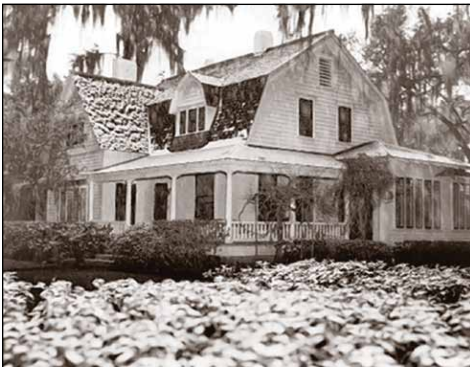
Snow on the roof of the Lock-Edwards home in 1958, one of 79 Dade City homes posted on fivay.org.
