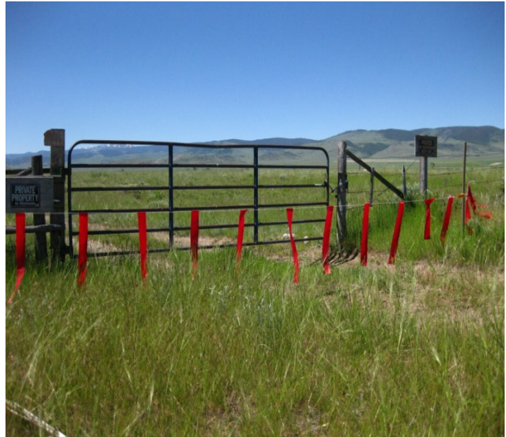
Figure 12: Fladry gate parallel to permanent gate. Both gates open from the right.
