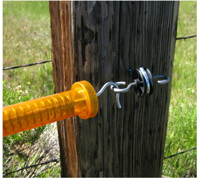
Figure 14: Gate handle connected to a wood post activator/insulator.
