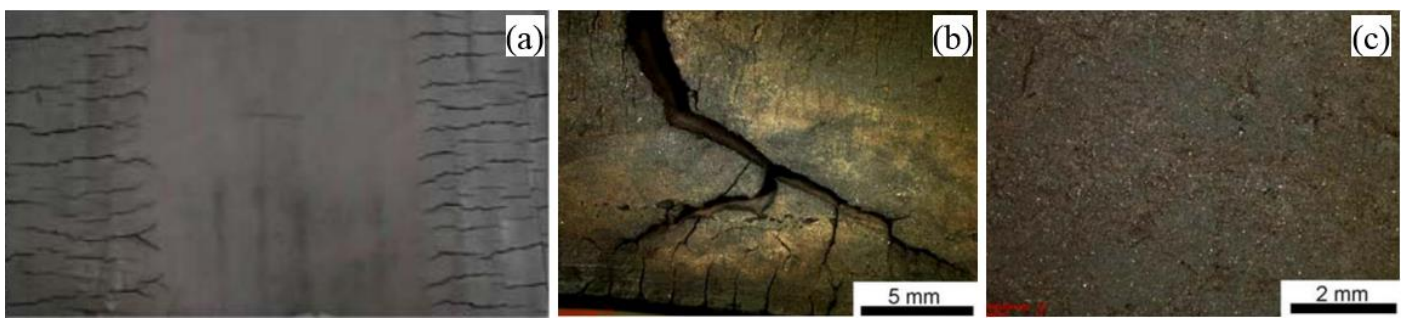
Figure 9: Wear of conveyor belt after eight years of service: (a) deep cracks in the rim region (b) Side view of a crack in the rim region, and (c) top view of the centre region (69).
