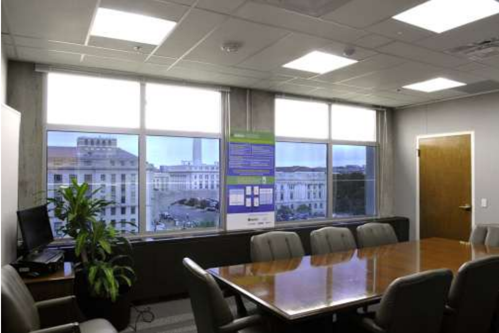
Fig. 1. Interior view of the conference room with upper and lower control zones.
