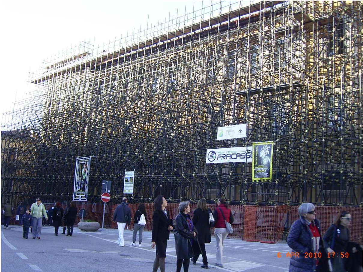
Fig. 7. Cordoned off area in the former business center of L'Aquila city (Italy). April 6th, 2010 (one year after the earthquake).
