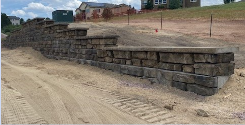
Pictured above are the completed project retaining walls.
