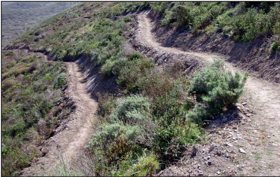
GRADE REVERSALS BEING USED TO CREATE INTEREST AND IMPROVE DRAINAGE
