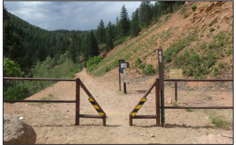
A USFS ACCESS GATE USED TO CONTROL TRAIL ACCESS
