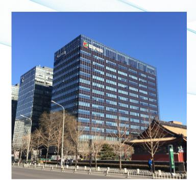
of 131 kWp in total. In 2018,the power generation of photovoltaic energy-saving curtain wall is 107,600 kWh,the annual power consumption of the building air conditioning and cooling system is reduced by 385,200 kWh,and the annual energy consumption of the building heating system is reduced by 357,200 kWh. In 2019,the power generation of photovoltaic energy-saving curtain
