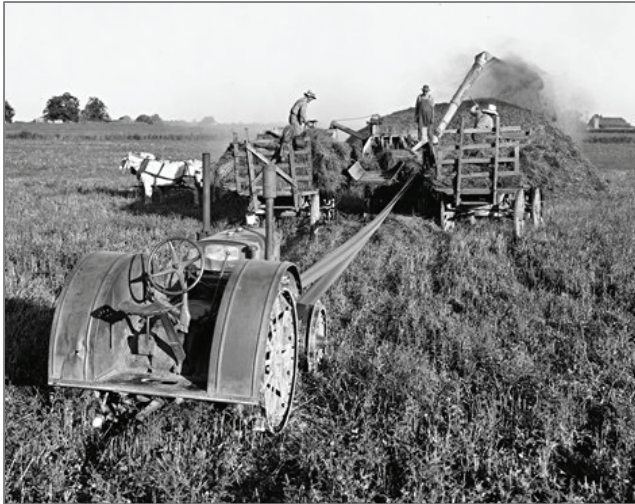
Figure 1. Tractor powering a belt-driven threshing machine from the 1920s.
