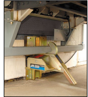
PHOTO 2: EXAMPLE OF A HOOK RESTRAINT SYSTEM
