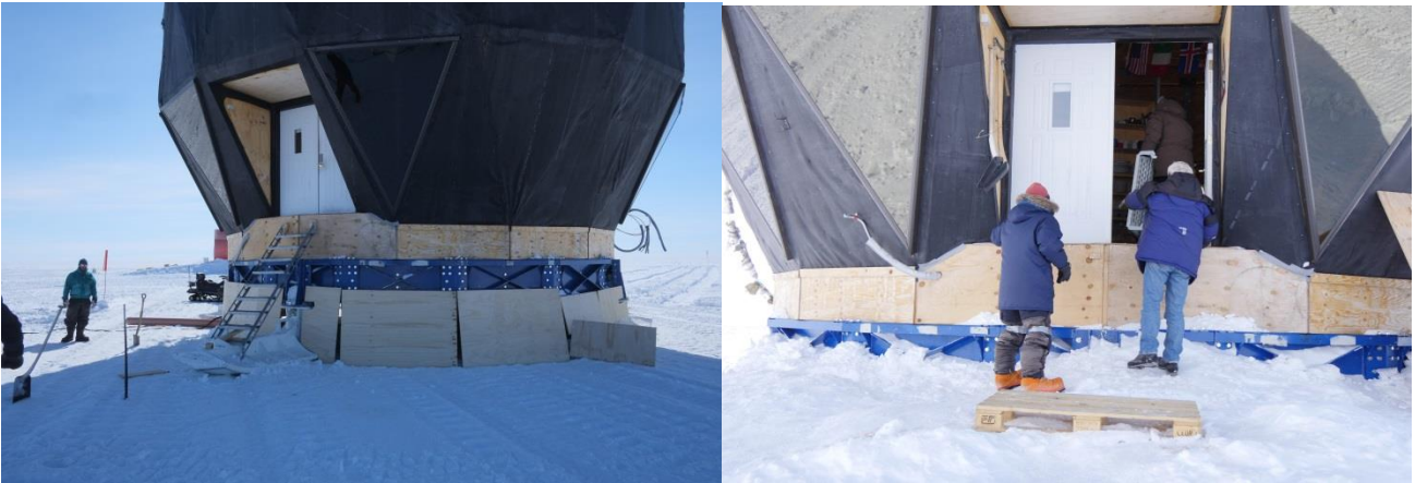
Left: The main dome at its parking position at EGRIP in June 2015. The undercarriage is covered by plywood before snow is packed around the base. Right: Photo from June 9 2015 just before the door is closed and crew leaves camp. Note the snow pack around the base.
