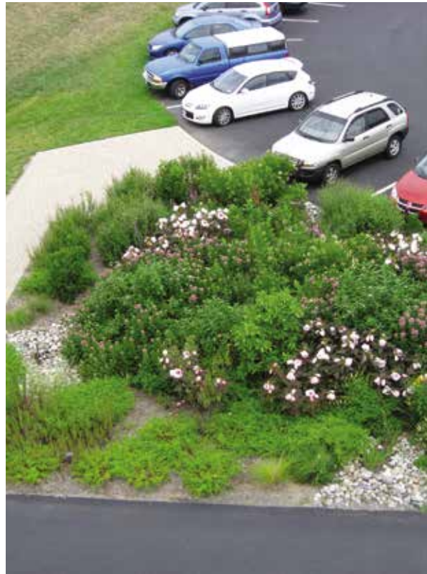
This rain garden at University of Delaware helps maximize resilience by reducing stormwater runoff from the pavement. Photo credit: University of Delaware Sea Grant
