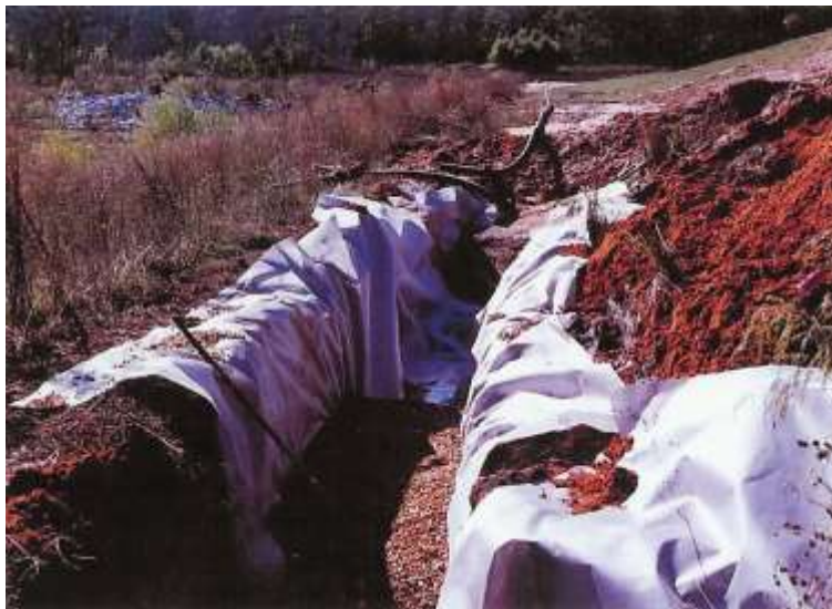
Figure 9. Typical Trench Drain Design Detail and Construction
