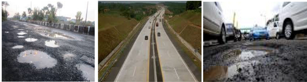
Fig. 2. The situation and conditions of road infrastructure.
