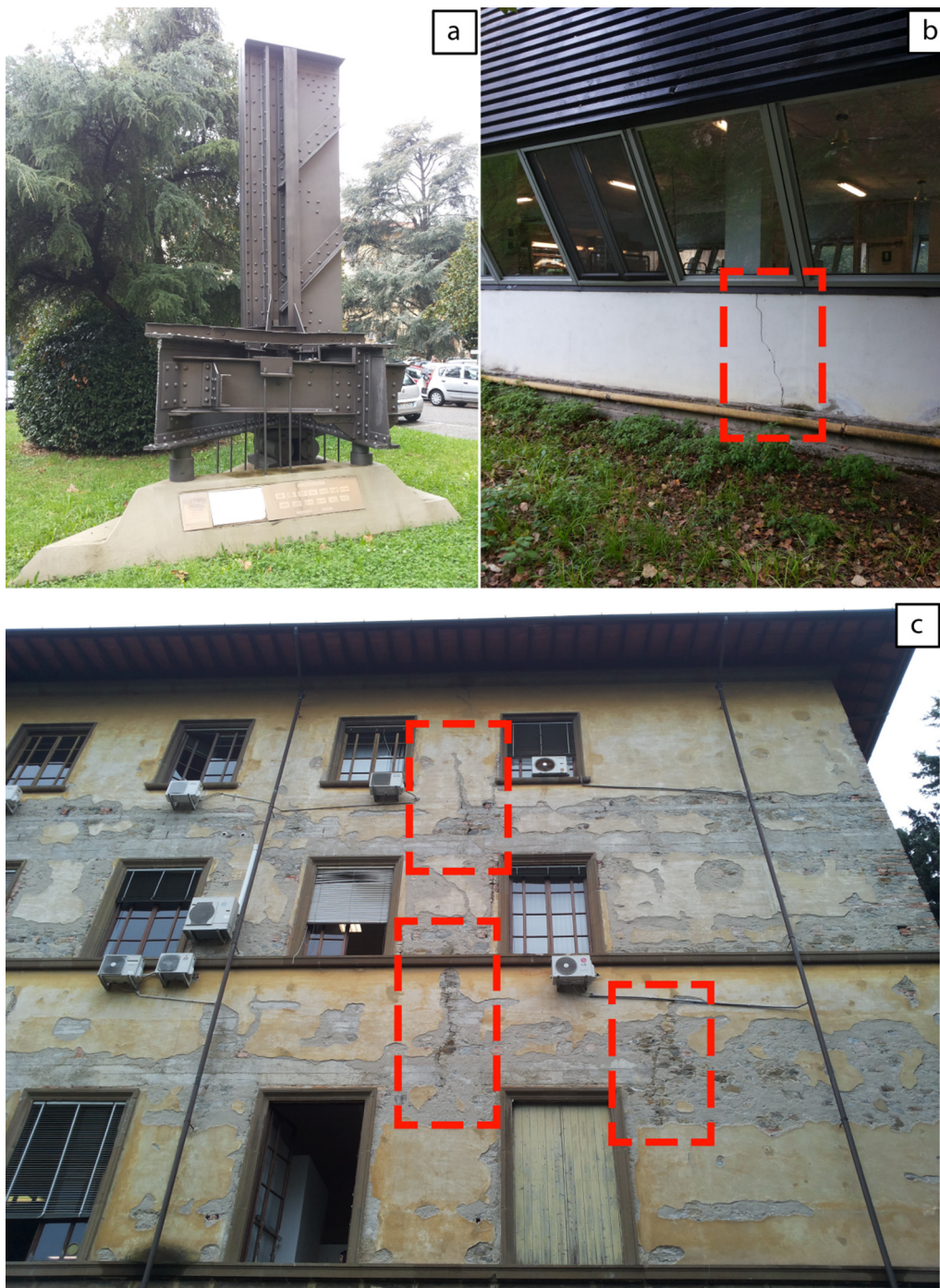
Fig. 8. (a) Contemporary sculpture installation, (b) façade of the canteen annexe and (c) the western façade of the main building of Santa Marta (photographs taken in October 2014) for which the ENVISAT ascending PS 2003–2009 show instability. Dotted red boxes in (b) and (c) mark major fissures running across the masonry and concrete structures. (For interpretation of the references to colour in this figure legend, the reader is referred to the web version of this article.)
