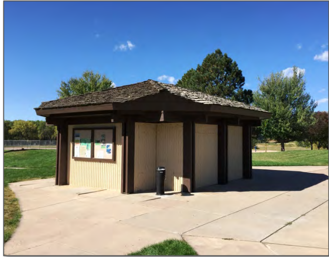
Figure 21 – Existing Restroom and Drinking Fountain
