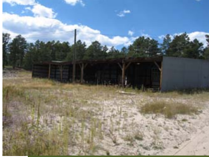
Ranch Shed to be Removed
