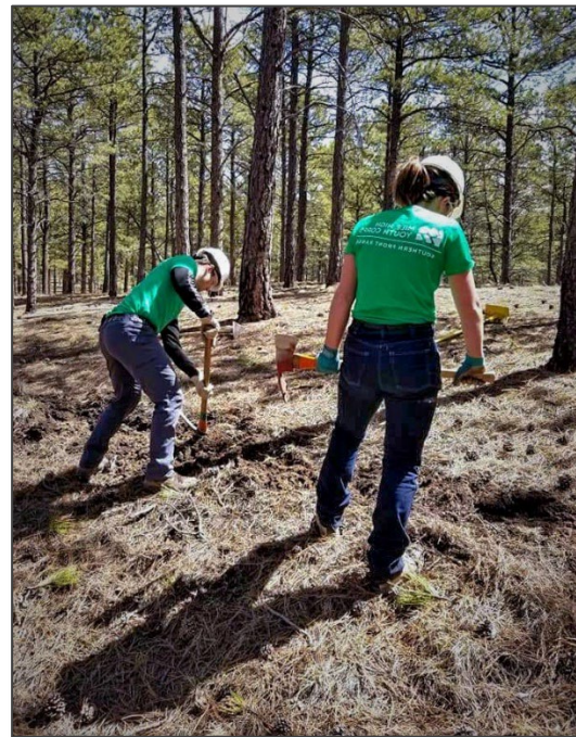
Figure 31 - Funded through a Great Outdoors Colorado (GOCO) Grant, Crew Members from Mile High Youth Corps Build Singletrack Trail by Hand in Pineries Open Space
