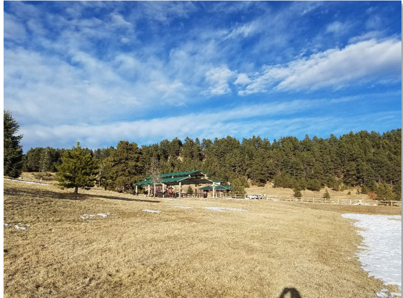
Figure 5 – Pavilion at Homestead Ranch Regional Park
