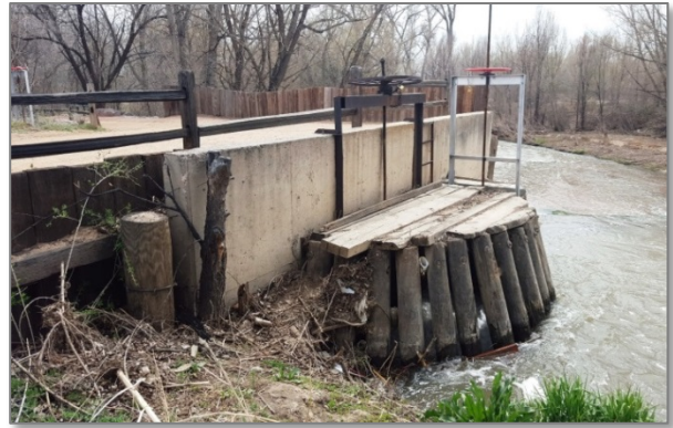
Figure 9 - Chilcott Ditch Headgate
