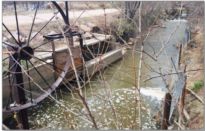
Figure 10 - Chilcott Ditch Diversion Structure
