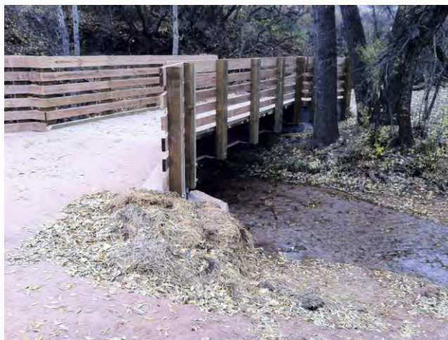
Pedestrian bridge across creek protects aquatic habitat
