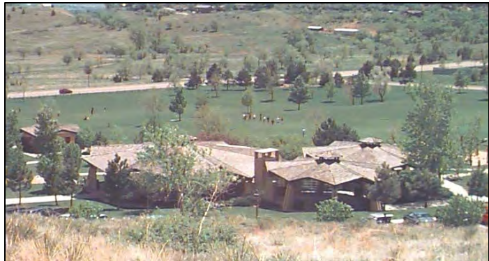
View of Pavilions at Bear Creek Terrace North
