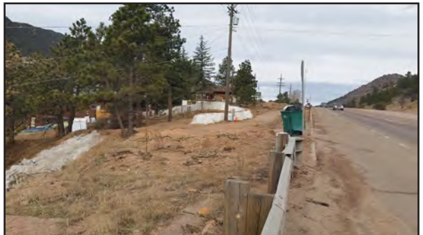
View of sediment build-up adjacent to U.S. 24
