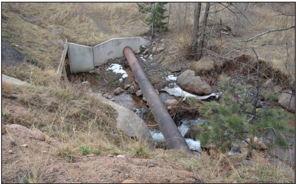
View of Fountain Creek. Place pedestrian bridge at Fountain Creek crossing
