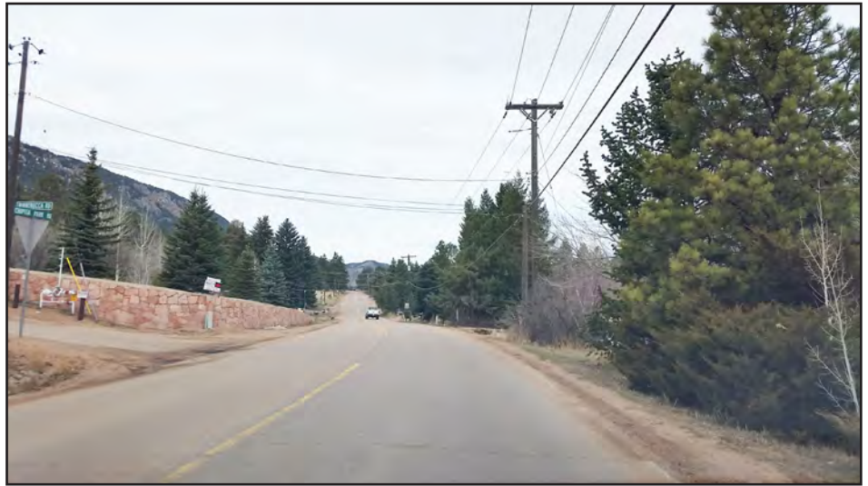
View of existing retaining wall at Winnemucca Road
