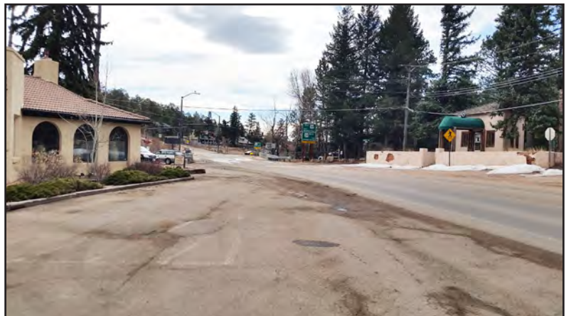
View of Fountain Avenue looking North
