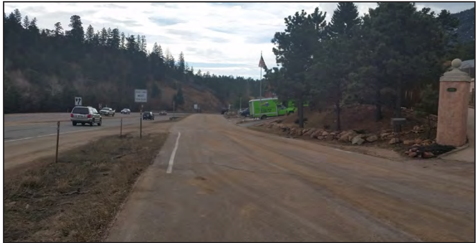
View of U.S. 24 frontage road. Place cross walk at vehicular access to U.S. 24
