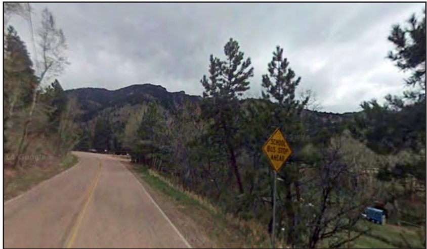
Example of Cut Slope Condition
