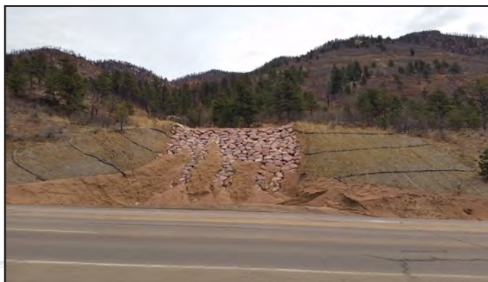
Fern Gulch Outfall After
