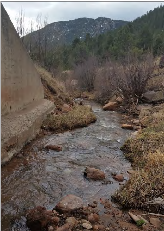
Fountain Creek south of Fountain Ave. looking east
