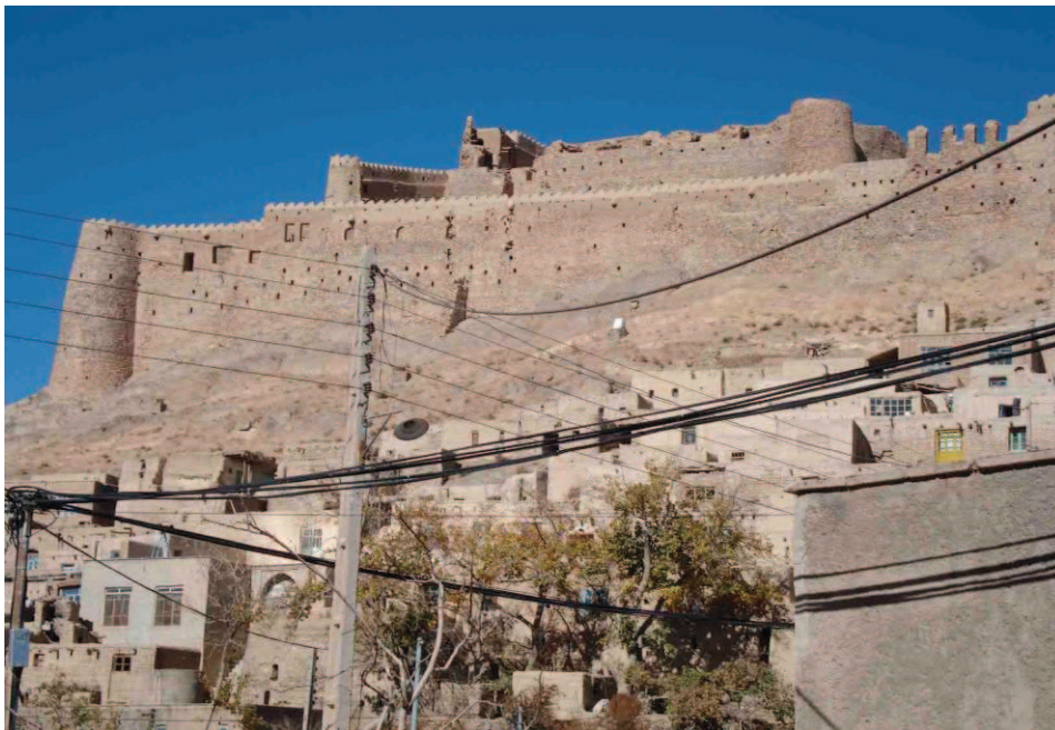
Fig. 11. Infrastructures of Telephone and Electricity for Tele-center in Forg village- Birjand.- East of Iran (Author, 2010)
