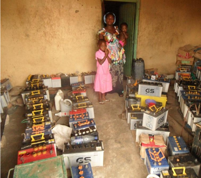
A battery charging station in a rural town of Uganda
