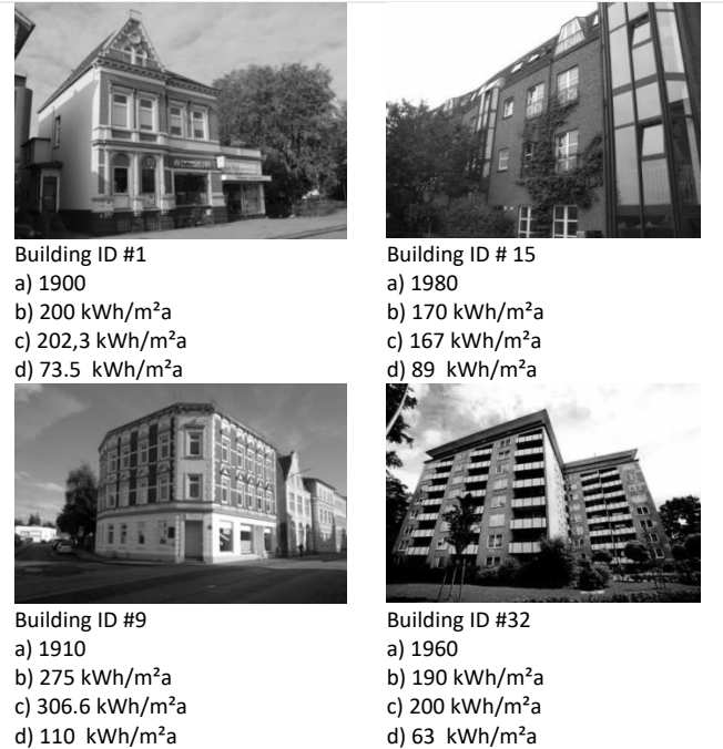
Figure 2: 4 Sample buildings from the building stock in the community with information about: a) Year of construction, b) Estimated heating demand after building cluster, c) Heating demand after energy pass d) Estimated heating demand after renovation.
