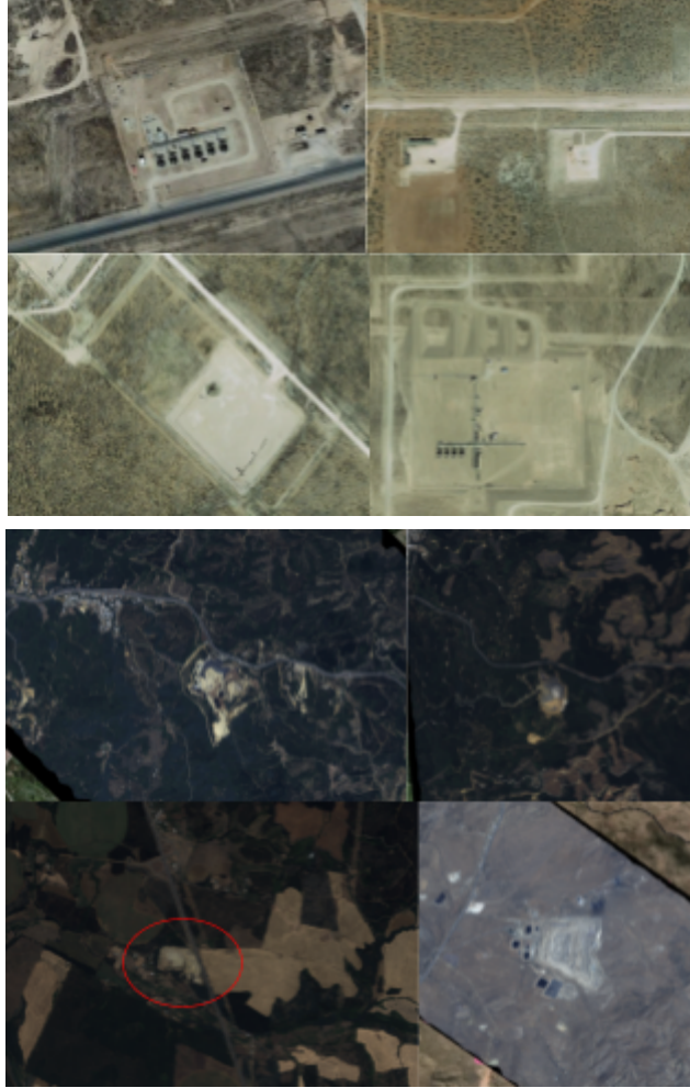
Figure 4. Typical aerial appearance of common infrastructure types known to be sources of CH 4 point sources. Top panel: Confined Animal Feeding Operations (CAFOs). Second panel: Surface coal mines and coal mine ventilation shafts. Third panel: Upstream oil&gas operations. Bottom panel: Solid waste management (landfills).
