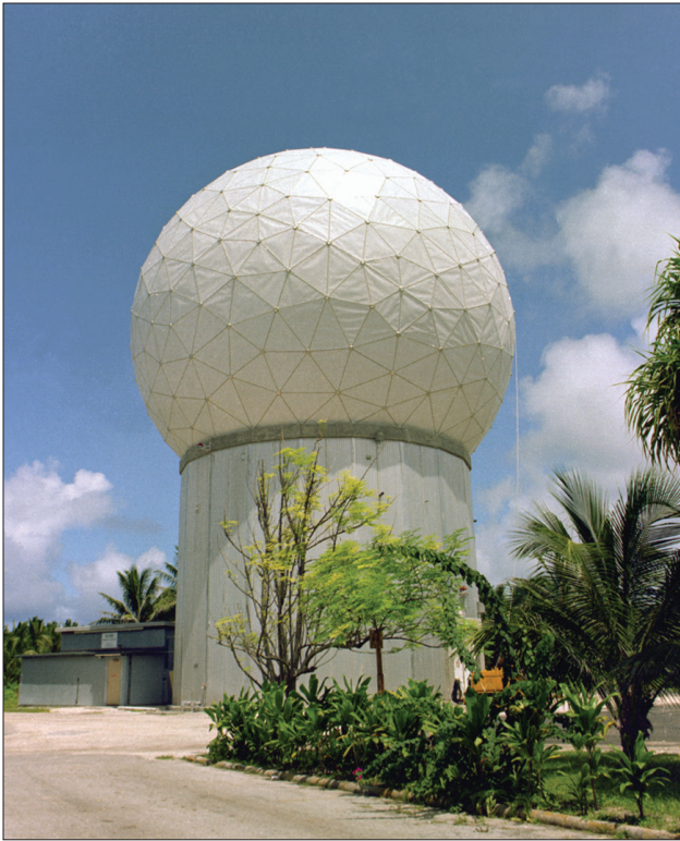
FIGURE 2. MMW is enclosed in a new Gore-Tex ® dome, which eliminates many of the issues associated with weather-related reductions in sensitivity.
