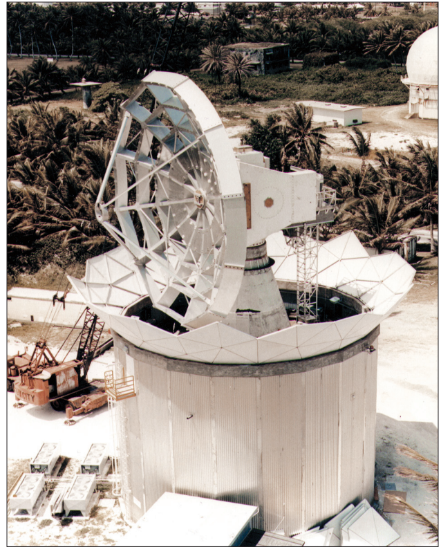
FIGURE 1. In 1983, the Millimeter-Wave Radar (MMW) was installed on Roi-Namur. Here, the radar is in place with initial components of the dome and antenna assembled.
