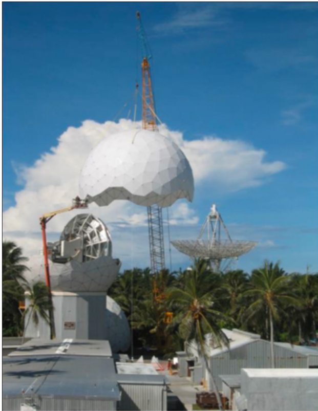
FIGURE 6. The MMW radome was replaced with Gore-Tex ® material to help eliminate issues related to water absorption. The image shows MMW undergoing radome replacement in 2003.
