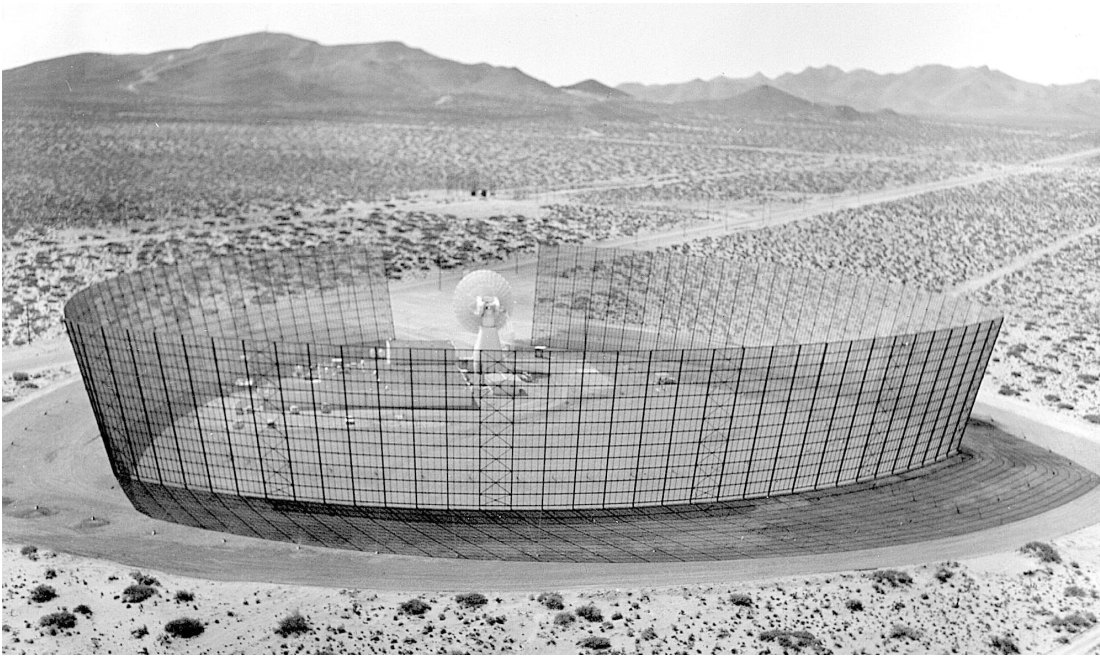
FIGURE 13. The ARPA Measurements Radar (AMRAD) with its clutter fence at the White Sands Missile Range, New Mexico (U. S. Army photograph). In this picture the 60-ft-diameter AMRAD antenna is aimed through a gap in the 104-ft-tall fence in order to work with radio-frequency (RF) calibration instrumentation on a boresight tower on a hill a few kilometers away. In actual missile-test operations the antenna is rotated about 180^\circ in azimuth and raised in elevation angle, its beam pointing over the fence at the incoming target complex. The fence keeps the antenna's sidelobes from illuminating the mountain ranges that border the Tularosa Valley, where AMRAD is placed, on its east and west sides. Before the fence was installed, strong clutter echoes from these mountains in the same range interval as the target complex made the collection of useful data difficult.
