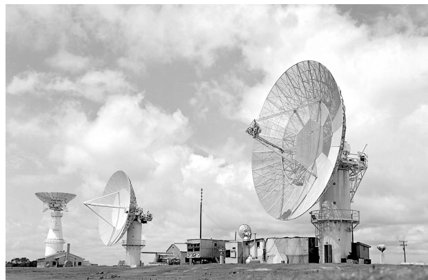
FIGURE 7. Radar antennas at the Lincoln Laboratory field site at Arbuckle Neck, Virginia, located near the Wallops Island, Virginia, launch facility. Site instrumentation consists of (from right to left) the S-band tracking radar, the multiplexed UHF and X-band cross-section measurements radar, and the SPANDAR (Space Range Radar) long-range trajectory and range-safety radar designed and built by Lincoln Laboratory for NASA.
