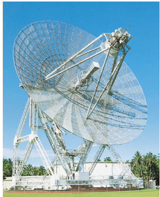
FIGURE 14. The ARPA Long Range Tracking and Instrumentation Radar (ALTAIR) on the island of Roi-Namur, Kwajalein Atoll, Marshall Islands.
