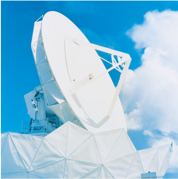
FIGURE 16. The ARPA Lincoln C-band Observables Radar (ALCOR) antenna and radome during installation on Roi-Namur. At C-band frequencies the forty-foot antenna provides a beamwidth of one-third of a degree, which is excellent for sensitivity and angular accuracy but difficult to point accurately.
