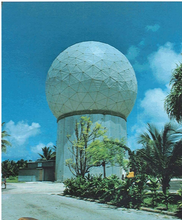
FIGURE 1. The millimeter-wave (MMW) radar at the Kiernan Reentry Measurements Systems facility on Kwajalein Atoll in the Marshall Islands. The radome protects the radar antenna from the corrosive island environment.
