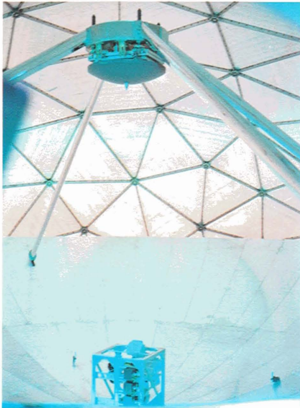
FIGURE 25. An inside view of the radome of the MMW antenna system, showing the BWG system at the vertex of the main reflector, and the subreflector with the dispersing cone at its center.
