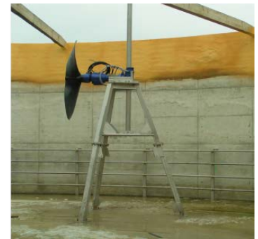
Submersible Mixers on a Freestanding Support Structure
