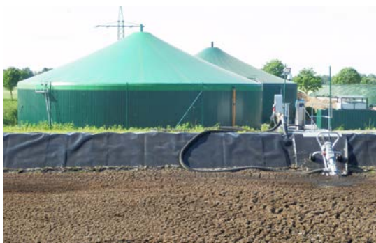
Digester with Center Pole Cover Support
