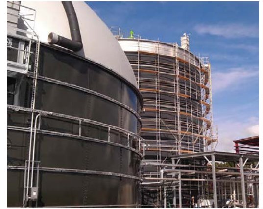
GenEarth – Berkeley County, SC (Charleston area)
