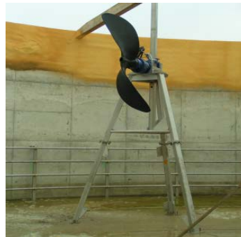
Submersible Mixers on a Freestanding Support Structure
