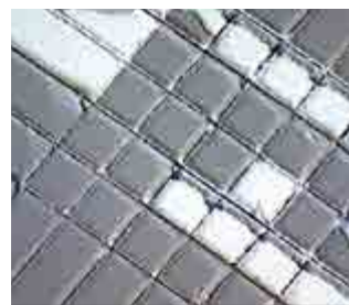
Loss of interlayer adhesion
