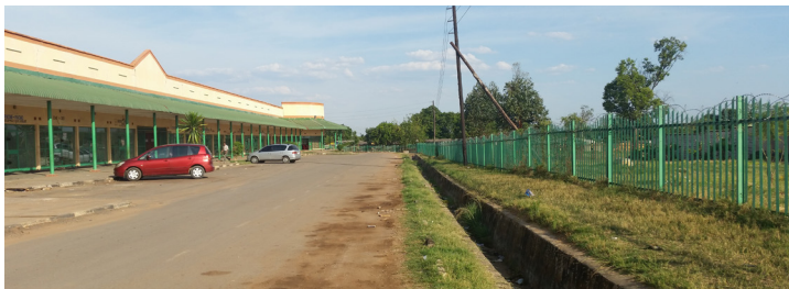
PHOTO NAKADOLI MARKET INFRASTRUCTURE, KITWE
